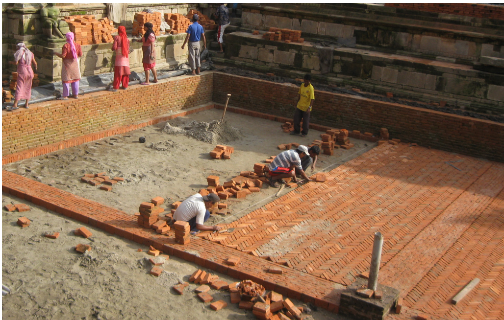
Top left: One layer of flat brick soling was placed above the mud. Bottom left: On-edge bricks on sand with lime surkhi pointing, were laid out in the historical pattern. Top: After completion.
