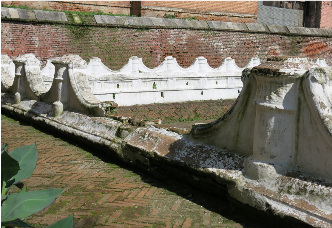
Left: Upper parapet, North. This is the only large section that is missing. Photo: Jan., 2013.
