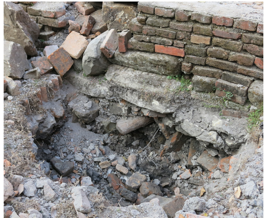
Left: The inner section of the platform was not properly built with brickwork, mostly filled with rubble. Photo: May, 2013 Bottom left: Excavation on south side of the platform. Bottom right: Detail of excavation. Below the pond surface, there were no proper foundation walls, only rubble mixed with stones. Photos: Jun., 2013.
