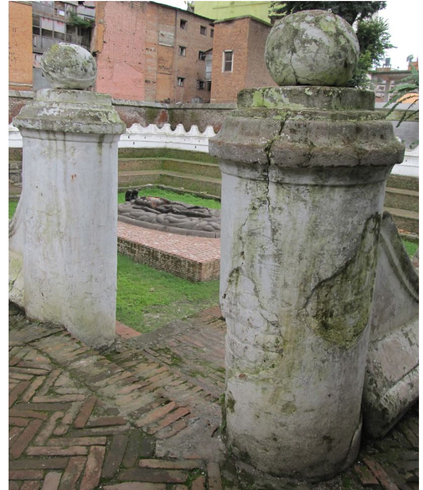
Right: North Entrance to the pond. Stucco plaster is broken off on the pillar and large vertical cracks are also visible. Recent repair work shows superficial beautification rather than the restoration of broken areas to increase the stability of the structure. The stucco plastered area was whitewashed and damaged elements were not replaced. Photo: Jul., 2013.
