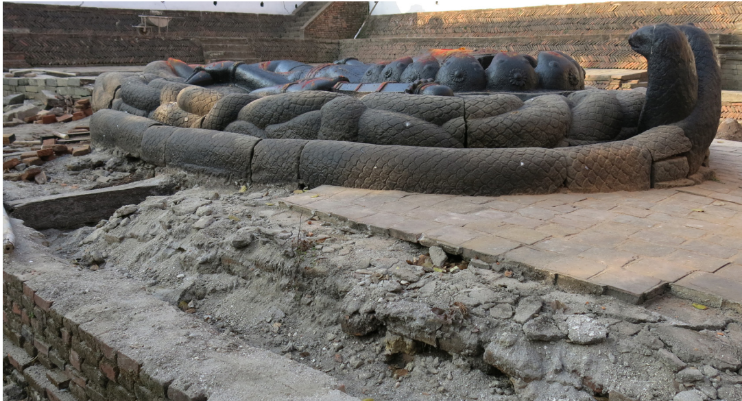
Left: The inner section of the platform was not properly built with brickwork, mostly filled with rubble. Photo: May, 2013 Bottom left: Excavation on south side of the platform. Bottom right: Detail of excavation. Below the pond surface, there were no proper foundation walls, only rubble mixed with stones. Photos: Jun., 2013.
