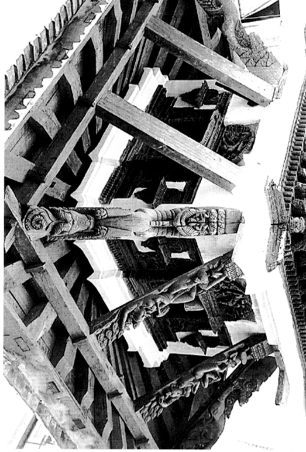
In situ comparative study of alternative solutions to the replacement of lost roof struts: plain timber props (right) and careful reproductions based on historical photographs (Photography by Mani Lama)
