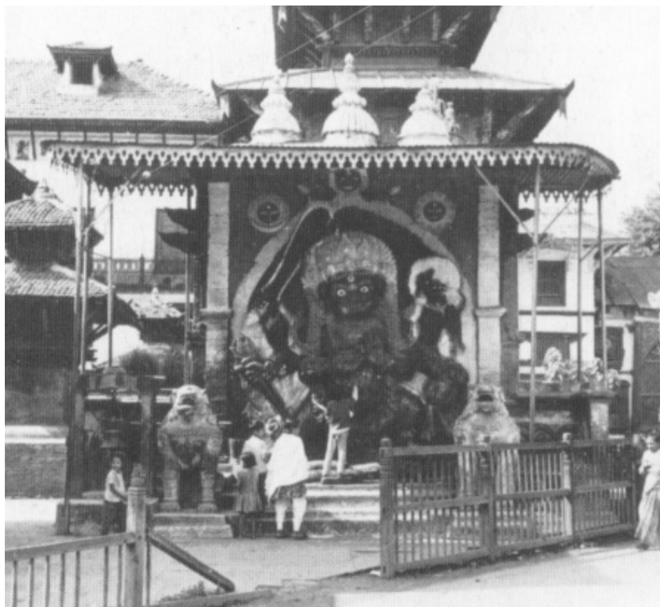
left: The roof structure with corrugated zinc sheets, supported by G.I. pipes was propped on top of the shrine. Photo courtesy: “Inventory of Kathmandu Valley: 1971”, published by UNESCO.
