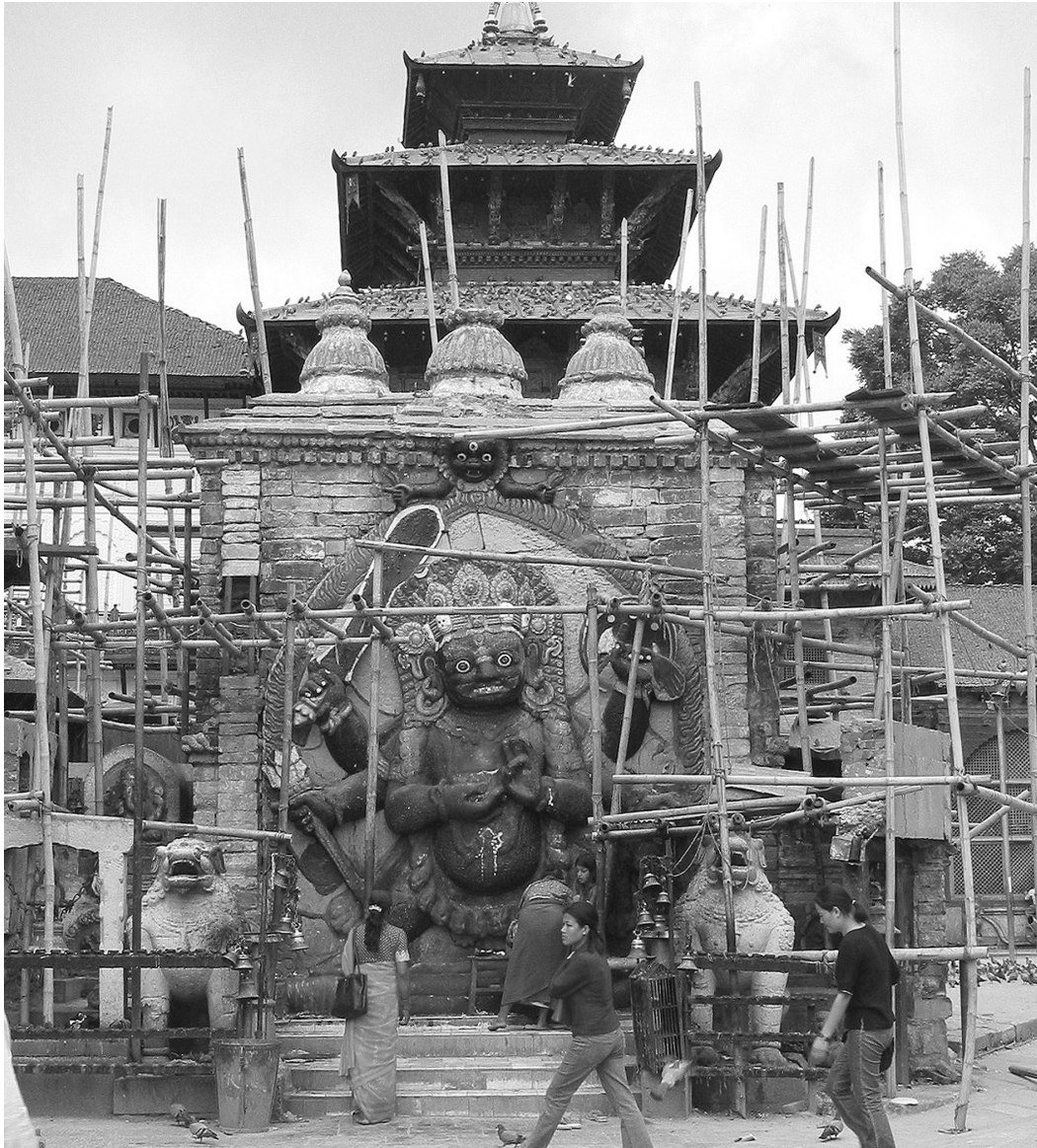
left: Much reduced and simplified version of the original structure was exposed when modern layers were taken off the shrine. Most of its significant details were either incomplete (pinnacle), reversed, damaged (cornice details) or lost (tympanum and the pillars). During the restoration, these details were recarved on the basis of the historical photographic documentation. Photo: Raju Roka, February 2004.
