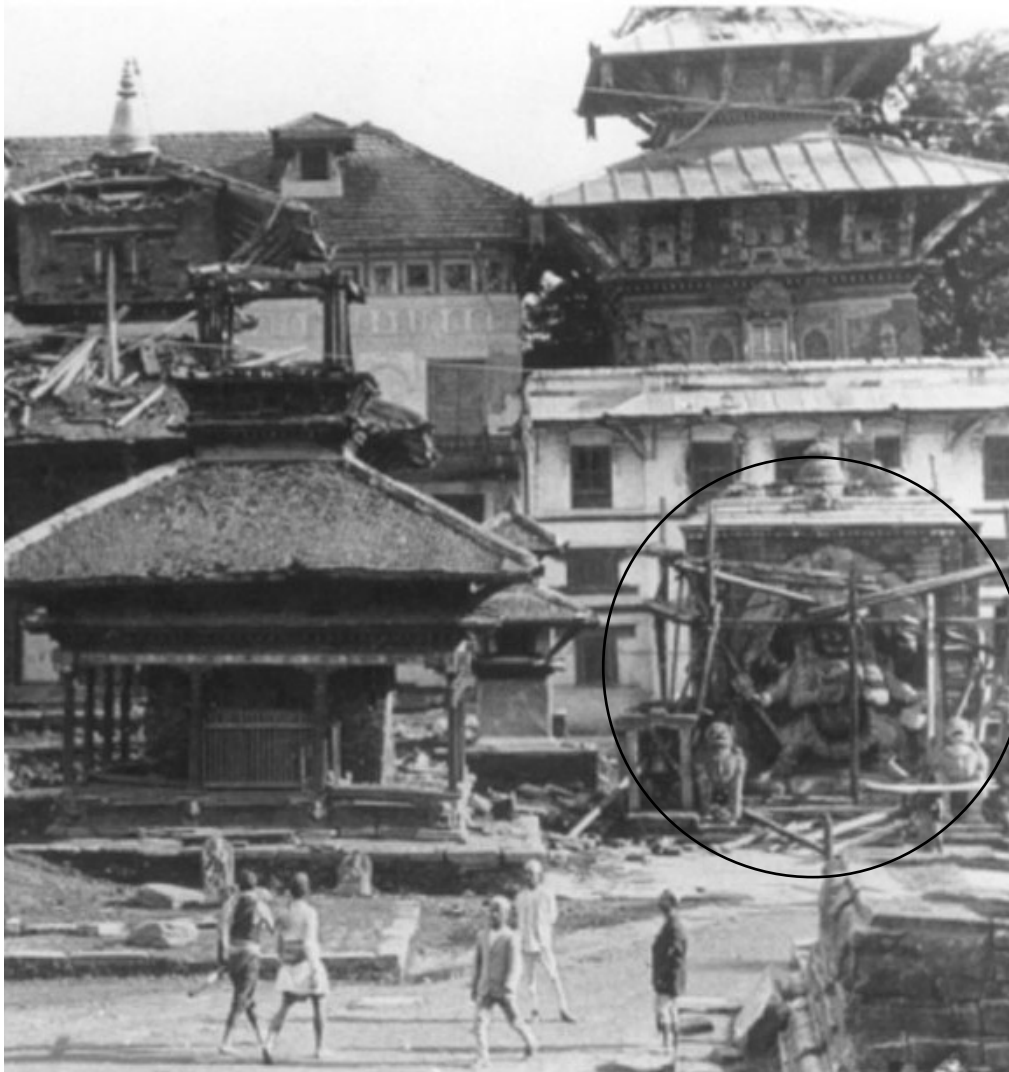
left: The great earthquake of 1934 devastated almost all of the temple structures in the Kathmandu Darbar Square. The upper level of the shrine including the cornice and the pinnacles had collapsed. This was not restored according to the historic configuration during the repair done in 1936, thus completely altering the original configuration of the shrine. Photo courtesy: Manju Rana.
