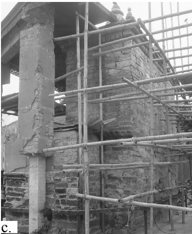
right: Removal of marble slabs and other recent layers revealed the extent of damage done to the shrine which we had not anticipated before. Much of the original fabric was found in poor condition and important details such as the tympanum was totally lost. Photo: Raju Roka, January 2004. above (clockwise direction): a. Kal Bhairav under scaffolding. b. The back wall had tilted 4" from the plumb line and the stone work was damaged because of cement used to fix the marble slabs and pre-cast cement blocks. c. Side wall after marble slabs were taken off. The modern additions also included the cement pointing on the joints. The wall was patched with cement plaster in many locations. Photos: Raju Roka, January 2004.
