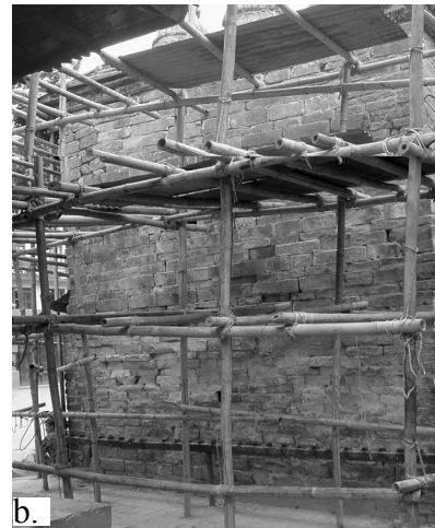
right: Removal of marble slabs and other recent layers revealed the extent of damage done to the shrine which we had not anticipated before. Much of the original fabric was found in poor condition and important details such as the tympanum was totally lost. Photo: Raju Roka, January 2004. above (clockwise direction): a. Kal Bhairav under scaffolding. b. The back wall had tilted 4" from the plumb line and the stone work was damaged because of cement used to fix the marble slabs and pre-cast cement blocks. c. Side wall after marble slabs were taken off. The modern additions also included the cement pointing on the joints. The wall was patched with cement plaster in many locations. Photos: Raju Roka, January 2004.
