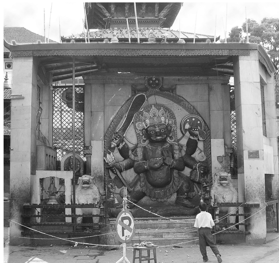
right: Kal Bhairav as it stood in December 2003, just before the commencement of restoration. The original form of the shrine was totally lost under the layers of votive offering donated to it. The marble clad concrete pillars supported the heavy metal roof above the shrine. Photo: Raju Roka, December 2003.
