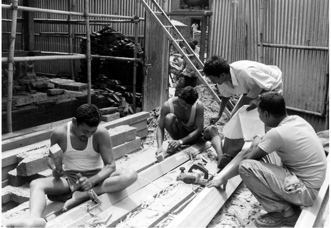
Carpenters work on plain timber fabricating rafters, purlin and wall plates.
