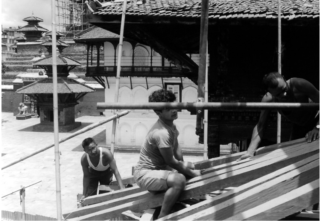
Carpenters installing the rafters on the lower roof.
