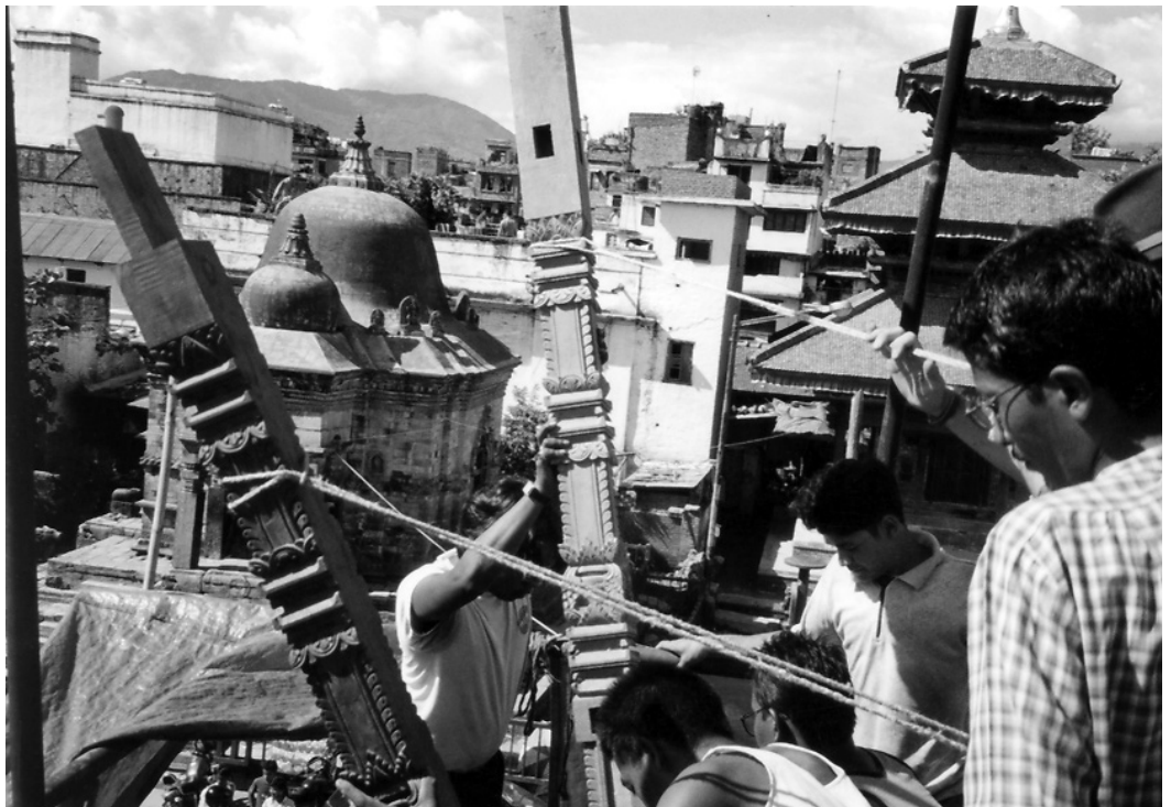
New carved inclined struts are in the process of installation on the upper tower.
