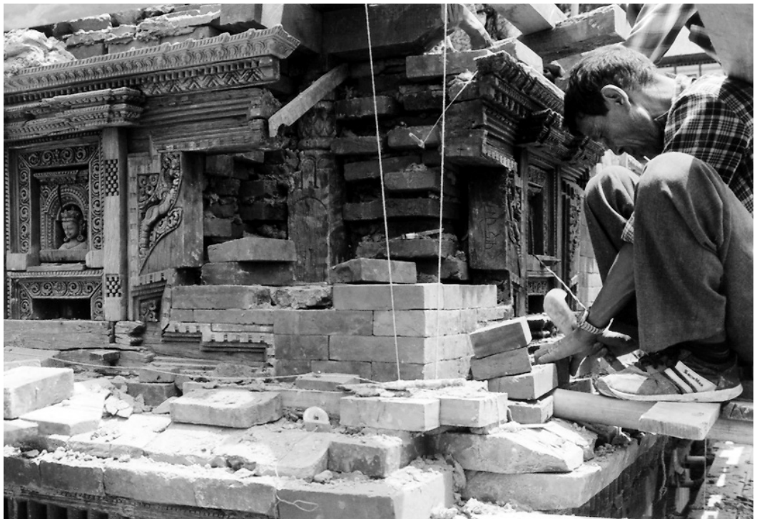
Rebuilding of the outer masonry wall on the first floor level in traditional brick ( dachi-apa and ma-pa ) incorporating the historical carved window.
