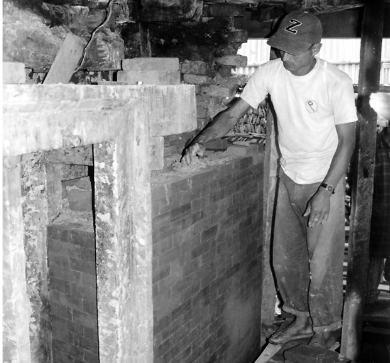
Rebuilding of a masonry wall on the ground floor sanctum with traditional brick ( dachi-apa and ma-pa ) which improves brick bonding.
