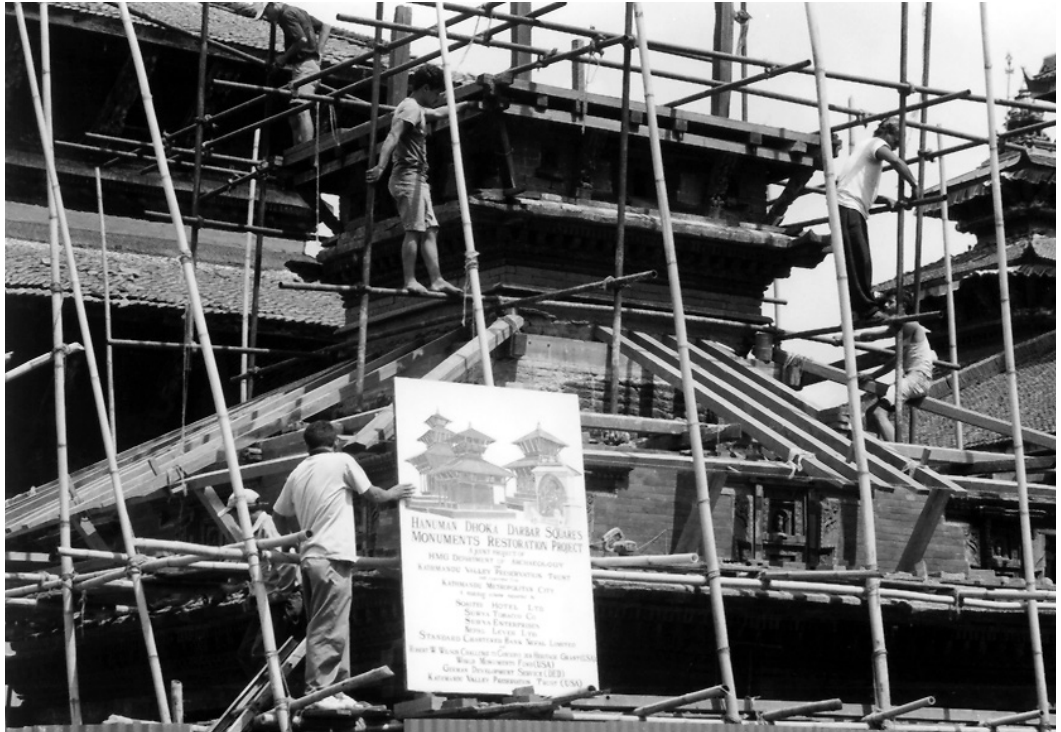
Upper tower dismantled to restore the historical figure.
