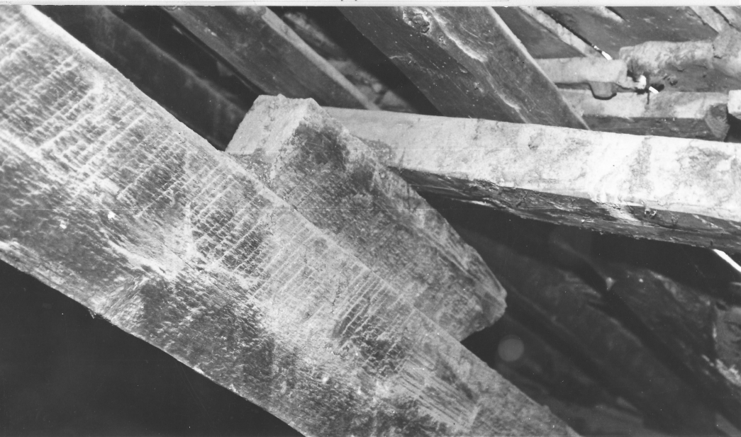
Support introduced between purlin and rafter
