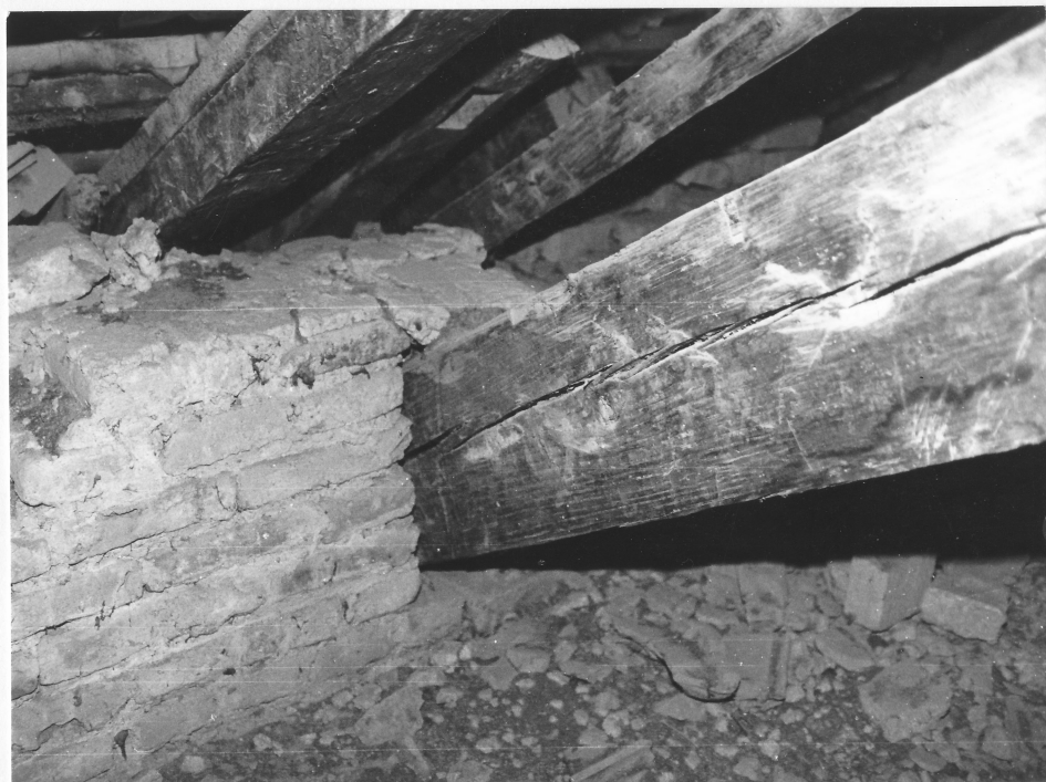
Truss' lower end hidden in low wall
