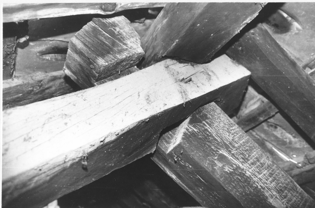
Roof details - ridge beam resting on truss
