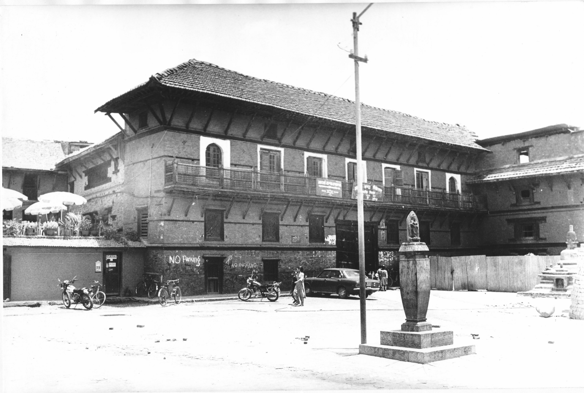
Patan Darbār – North Wing
