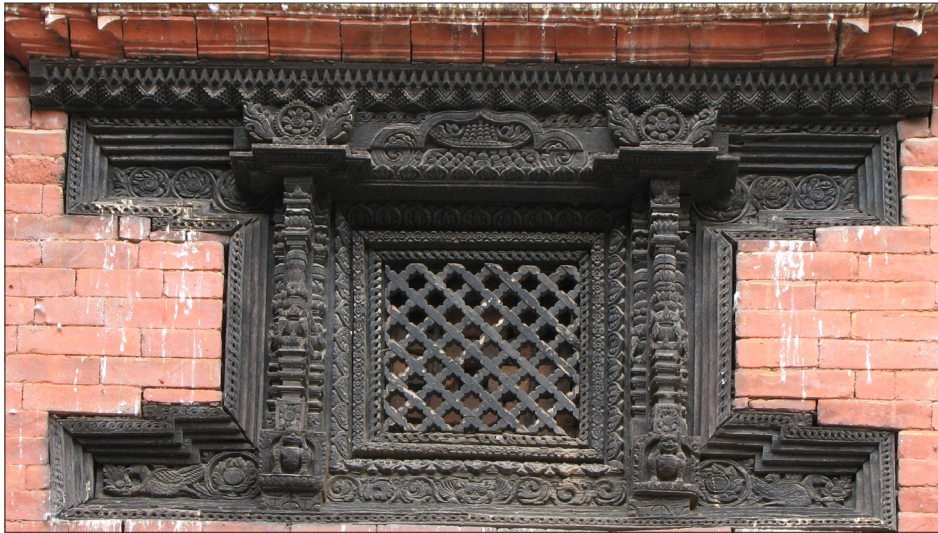
2.8.W.02 Frame-original, Lattice-new
