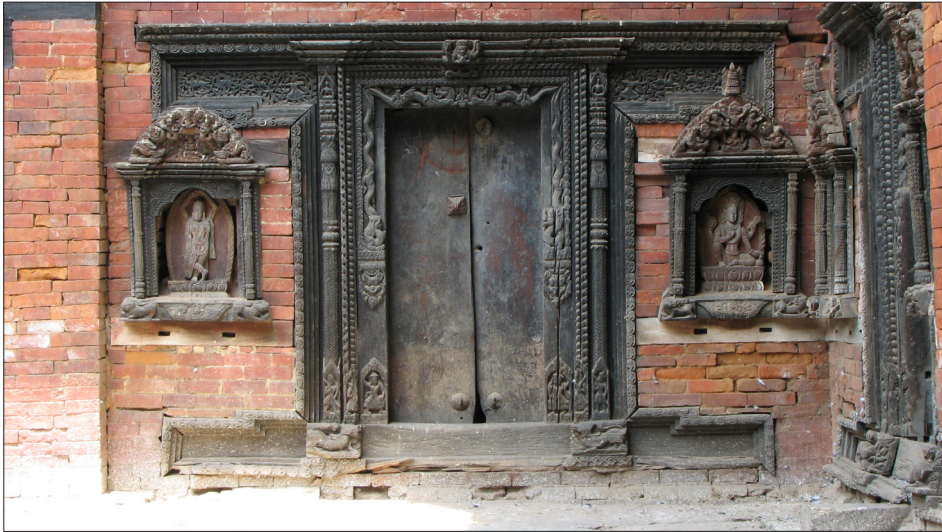
2.5.D.02 Door frame-original / authentic, Shutters-original
