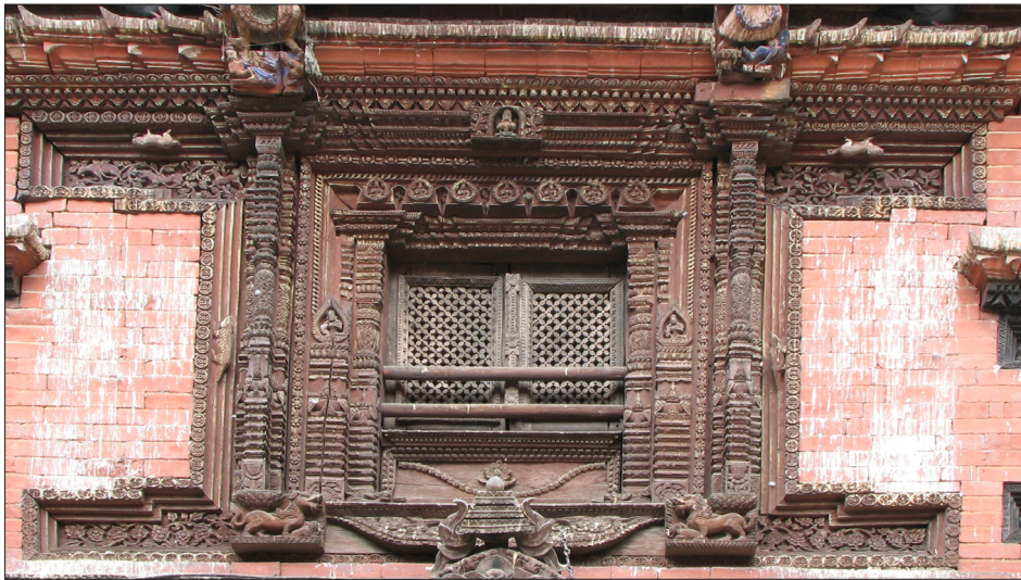
2.8.W.03 Frame-original /authentic, Shutters-new (added in 1990s)
