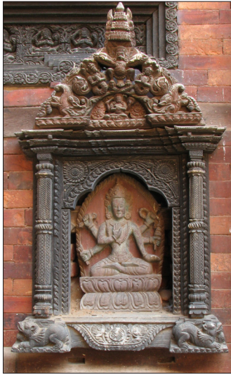
2.7.N.02 Tympanum-original, frame-after the earthquake, statue-after 1988
