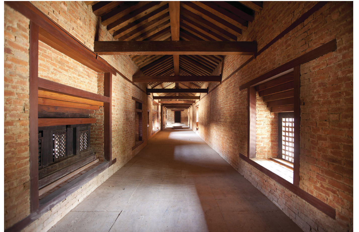
Gallery 01 before completion of wall plaster and tile floors. Photograph by Kishor Kayasta, December 2011
