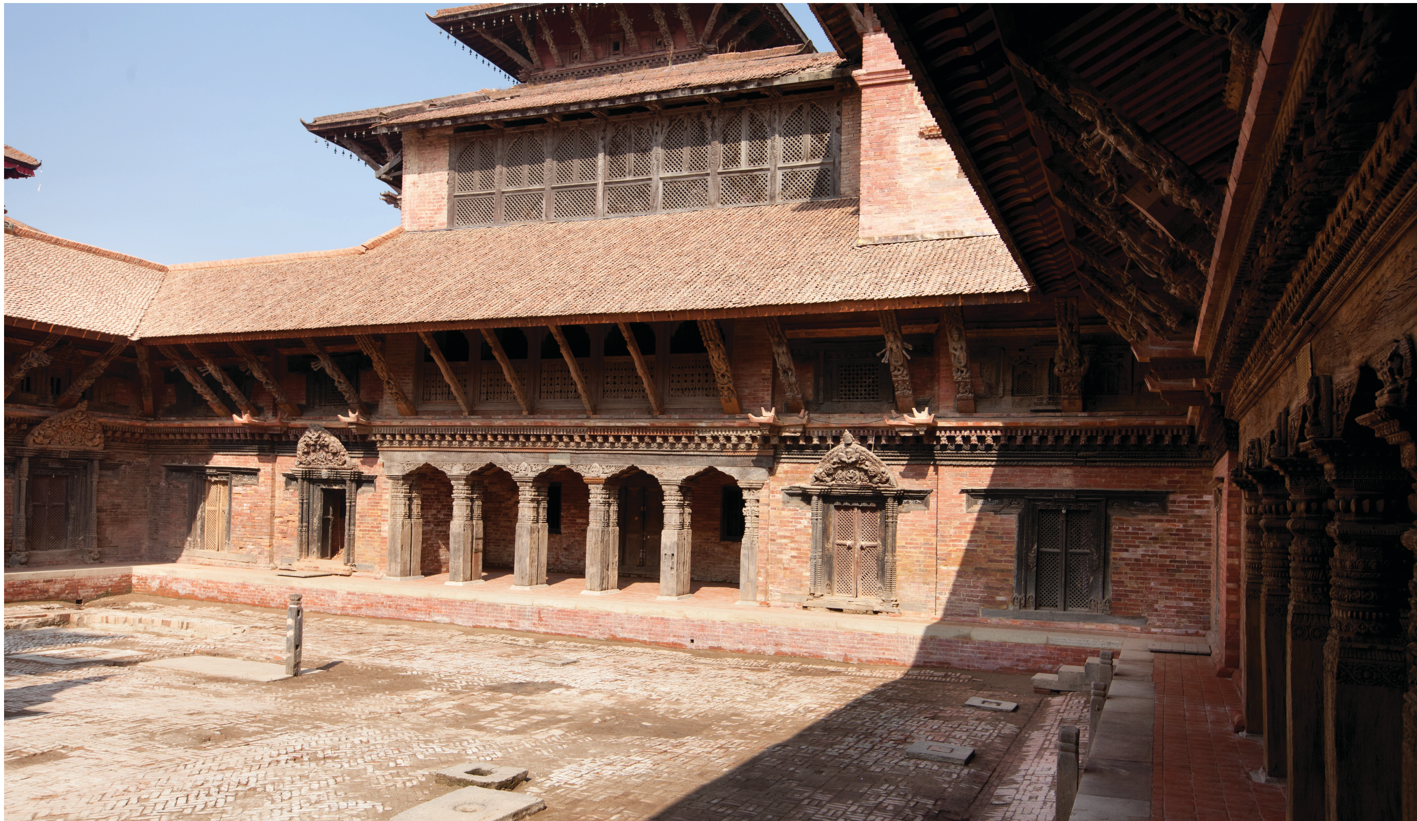
Mulcok North Wing - after restoration Photograph by Kishor Kayasta, December 2011
