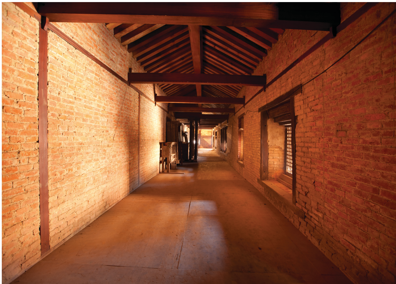
Mulcok East wing interior - after restoration, installation of tile floors and wall plaster pending Photograph by Kishor Kayasta, December 2011
