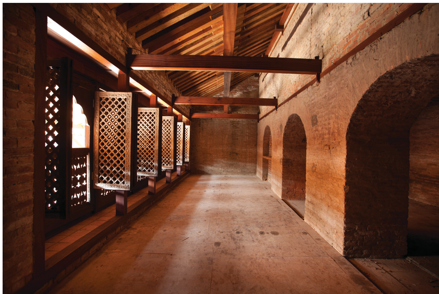
Mulcok north wing interiors after restoration (tile floors and wall plaster remaining to be done) Photograph by Kishor Kayasta, December 2011
