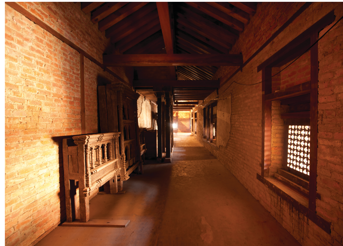
Mulcok South wing interior - after restoration, installation of tile floors and wall plaster pending Photograph by Kishor Kayasta, December 2011
