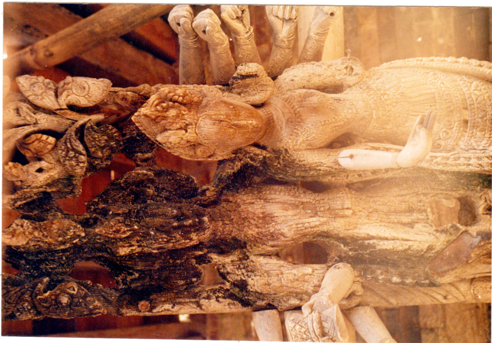
LOWER ROOF STRUT 107: DOCUMENTATION OF MILDEW AND WET ROT, MARCH, 1992.
