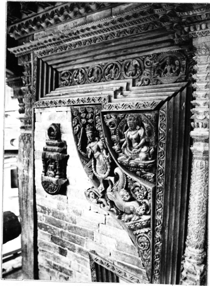
SPREAD TIMBER JOINTS AT BASE STORY. LEFT: NORTH ELEVATION, LEFT SIDE. RIGHT: CORNICE AT NORTHWEST CORNER.
