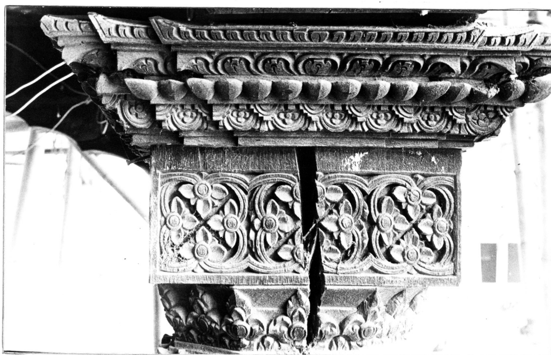
VARYING FLORAL MOTIFS ON TWO ADJACENT PILLAR CAPITALS: NORTHWEST CORNER.
