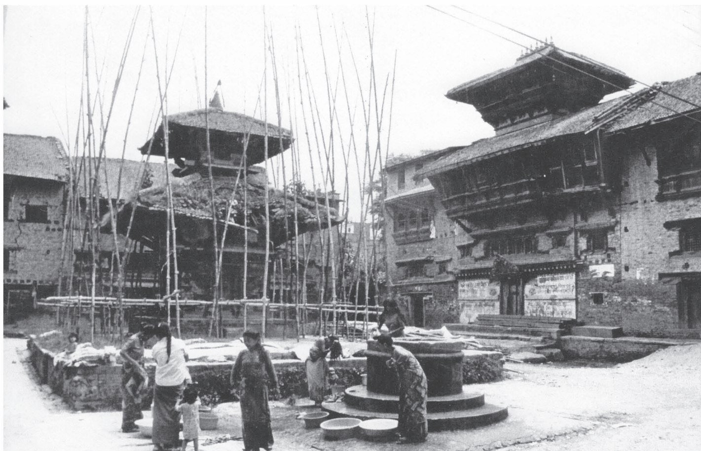
Scaffolding on the temple by Sulima Guthi. Photo: 1994.
