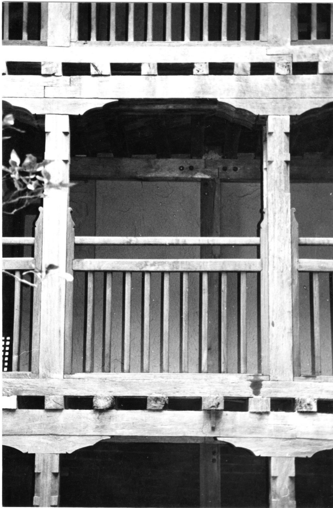
Courtyard elevation (west) after restoration showing rebuilt gallery incorporating four historical timber posts with new "feet".
