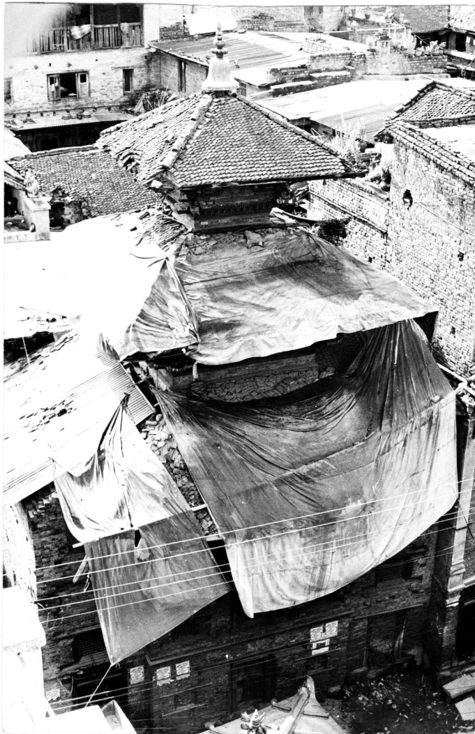
Pre-project activities SE view after emergency tarpaulin cover on the roof to protect from monsoon rain, 1992.
