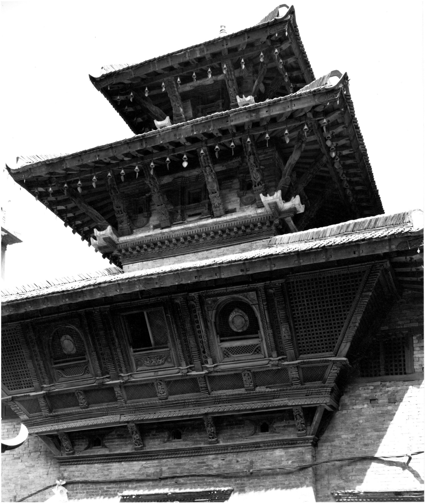
After restoration Upper levels of main facade after restoration. Photo: John Hall, May, 1997.
