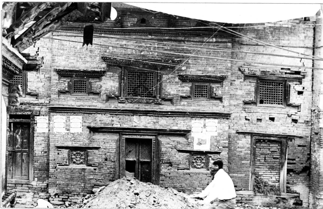
Front facade, lower two stories. April 1993
