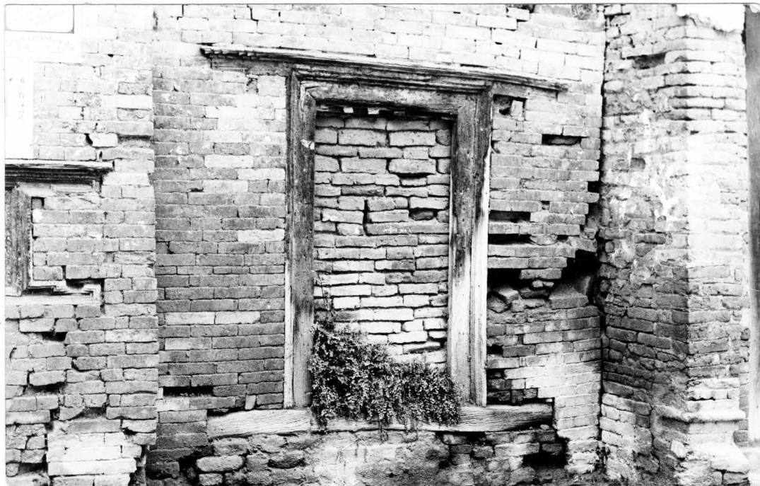
Above : New opening front facade left, from 1977 repairs.
