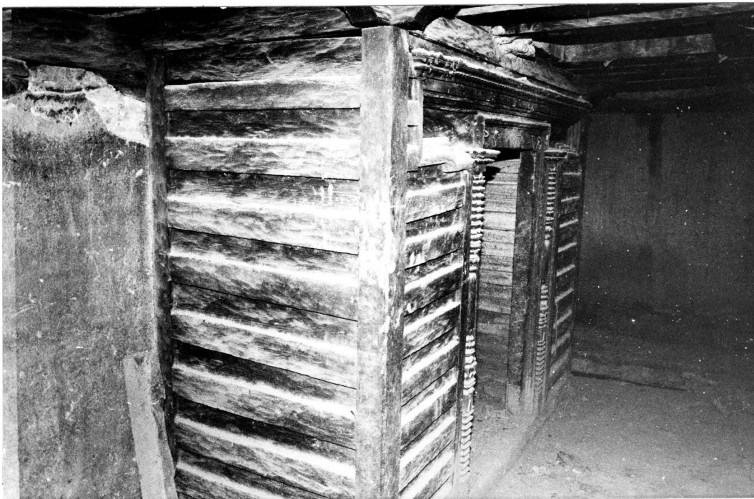
Timber partitioned esoteric shrine, second floor.
