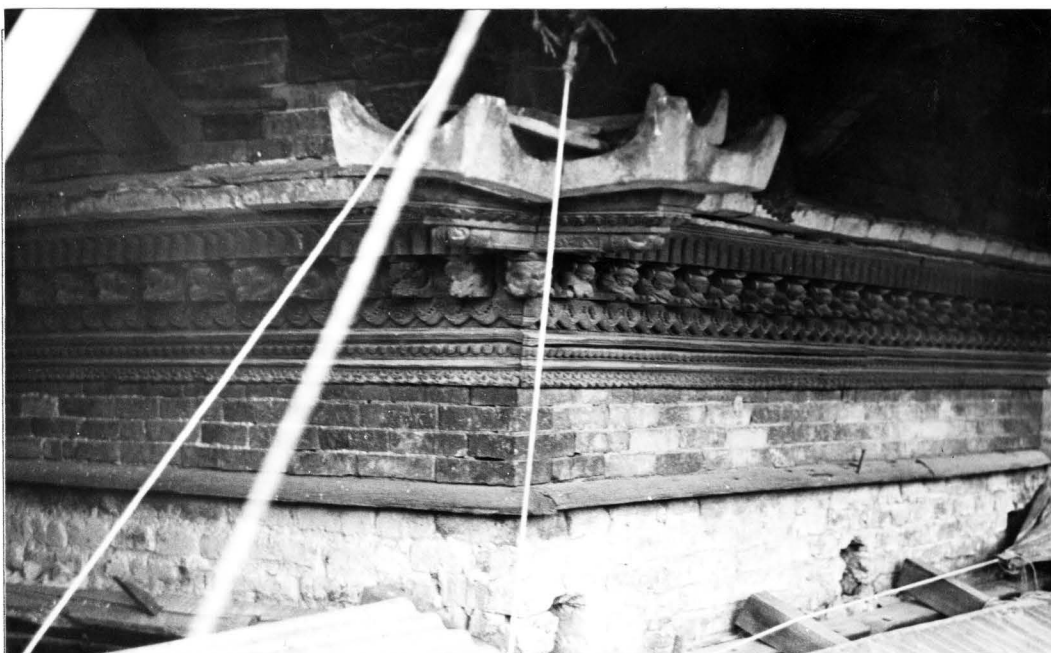
Upper level of rooftop pagoda shows daci apa framed by timber cornice pieces. Below common fired brick with visible mud mortar joints. All in excellent condition.
