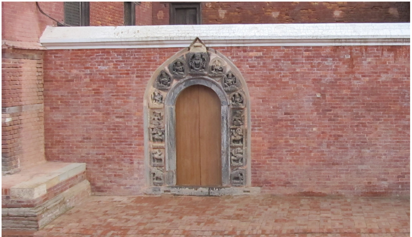
April 2008, November 2012: South stone gate before and after restoration. The inner courtyard will be part of the future Architecture Galleries at Mul Chowk.
