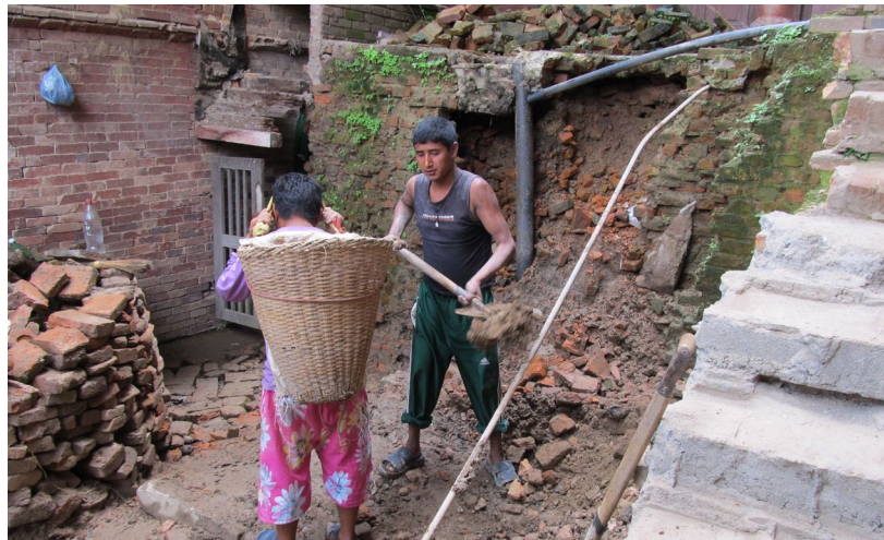
July 2012: Debris being removed after excavation of the pavement.
