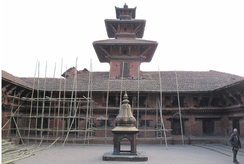
February 2010: The restoration project began by building scaffolding.
