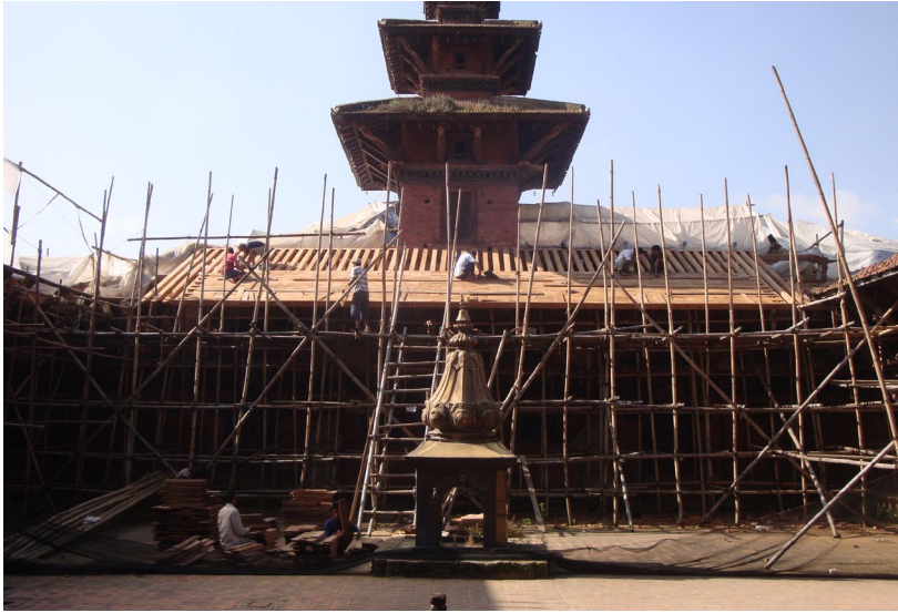
January 2011: Installing hardwood and plywood planking on the timber joists of the south wing.
