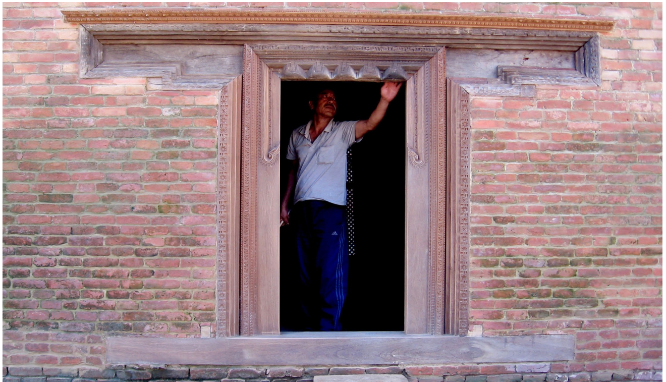
February 2007, October 2010: An existing east wing door-frame that had fallen into disrepair was repaired, reusing as much of the historical timber elements as possible. The doorway is shown here before and during restoration period.
