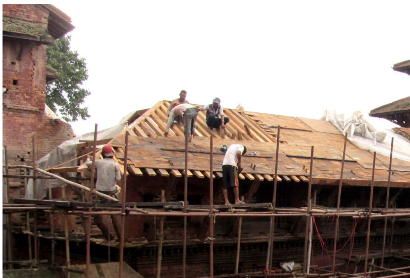
September 2011: Uniting roof timber elements on the northwest corner.
