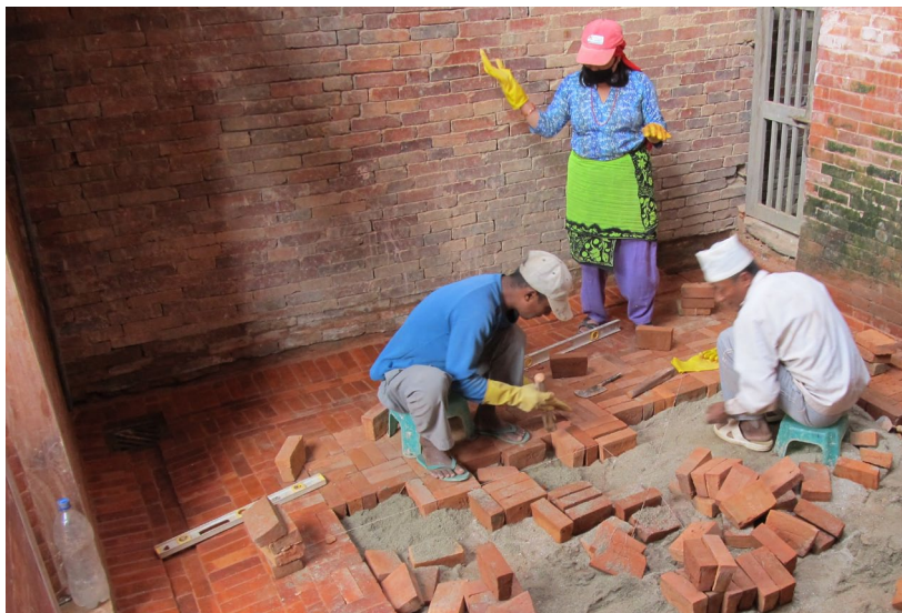
November 2012: Installing brick on-edge paving in the courtyard.
