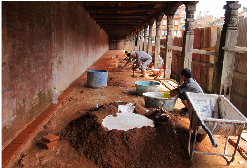
August 2012: Installing chikah-apa floor tiles over lime and brickdust ( surkhi ) mortar.
