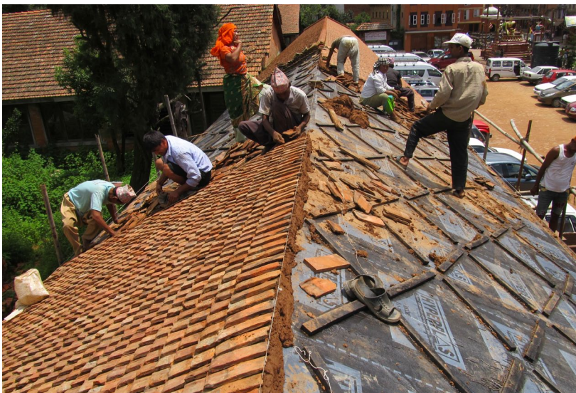
August 2012: Application of traditional terracotta ( jhingati ) roof tiles above a mudbed on a waterproof membrane.
