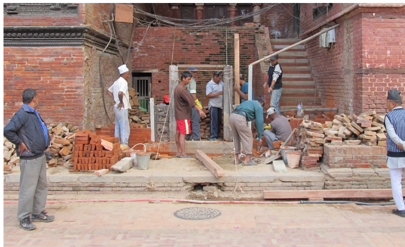
October 2012: Building the brick wall surrounding the gate using traditional ma-apa brick in lime surkhi mortar.
