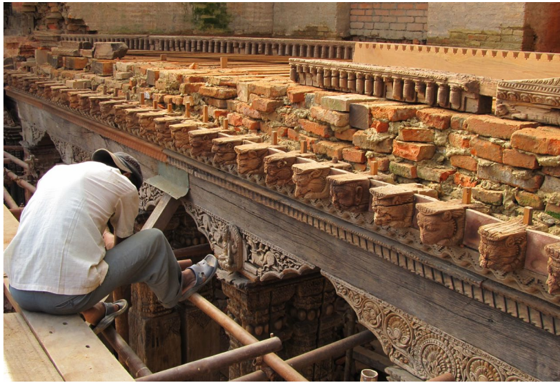
July 2011: The lion heads on the timber cornice were cleaned and reinstalled.
