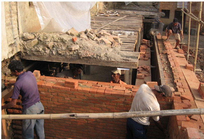
June 2011: Rebuilding the partition wall on the east wing ground floor using traditional ma-apa bricks in mud mortar.
