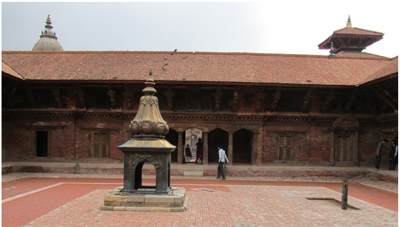
December 2012: Views of west wing's west (exterior) and east (courtyard) façade after restoration was completed.
