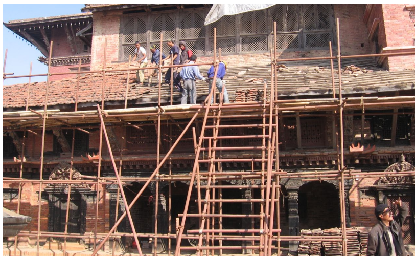
August 2010, March 2010, January 2011: Removing the existing roof structure from the east, south and north wings.
