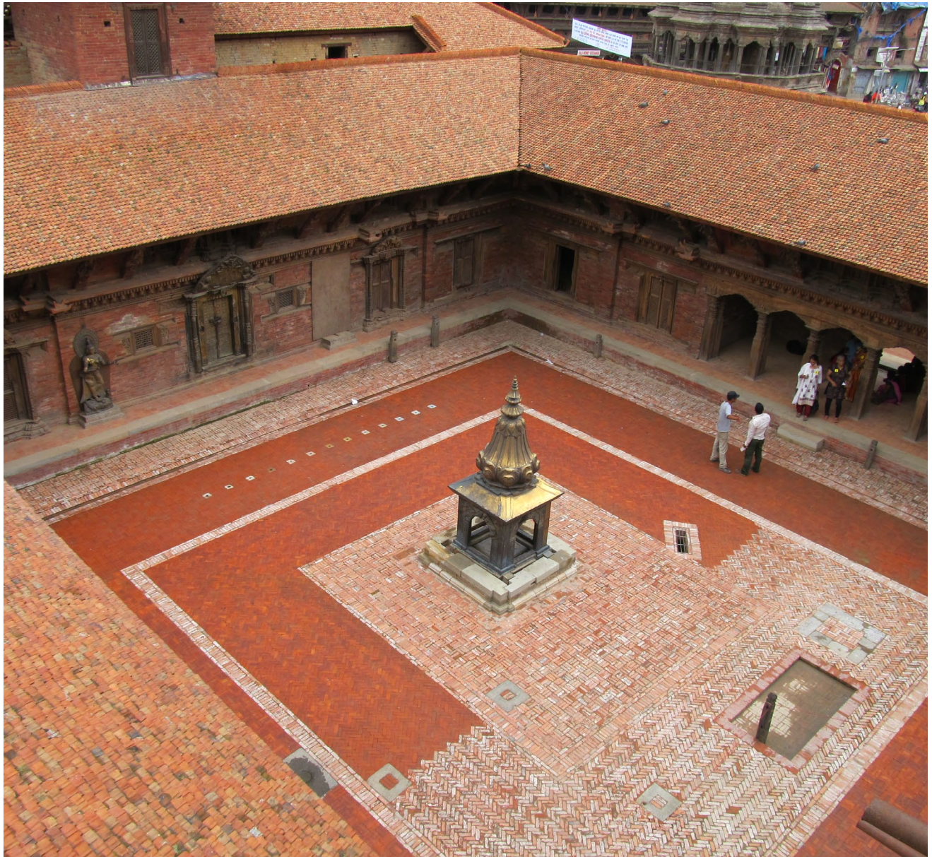
June 2012: Courtyard shortly after complete restoration. The redder bricks are newly made custom bricks and the rest are existing historical bricks that were reused.
