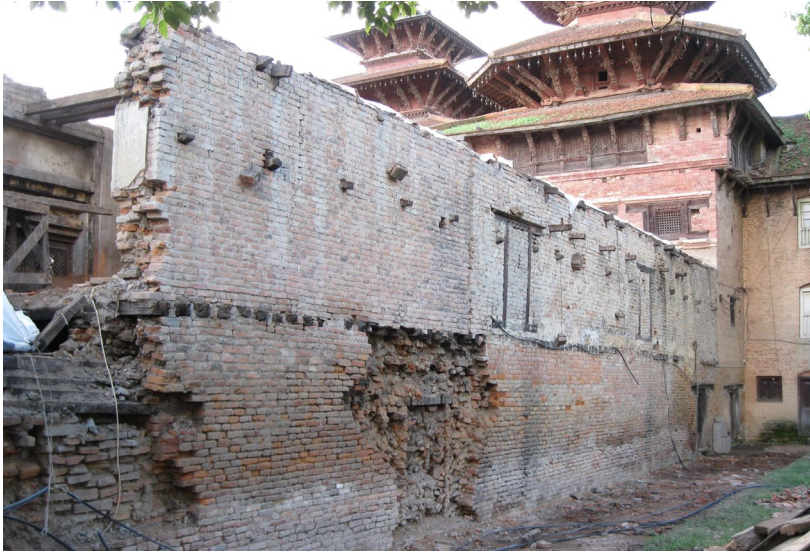
May 2010: East wing brick wall during deconstruction.
