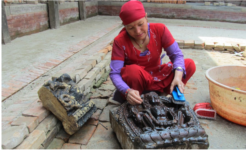
March 2012: Woman cleaning a stone element of the gate using acetone.
