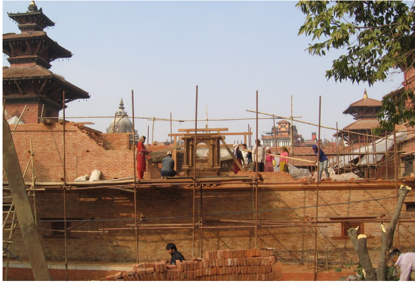
June 2011: Reconstruction of the east wing façade.
