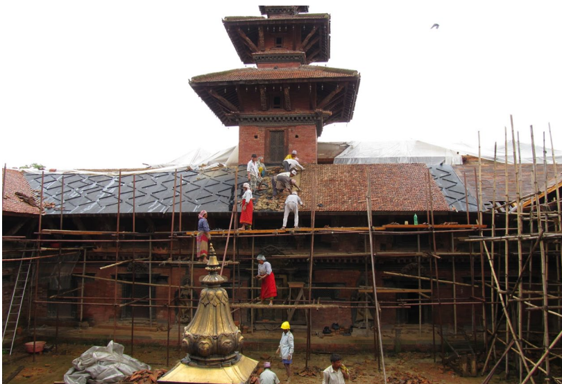
July 2011: Installing jhingati roof tiles over a mud-bed on a waterproof membrane.
