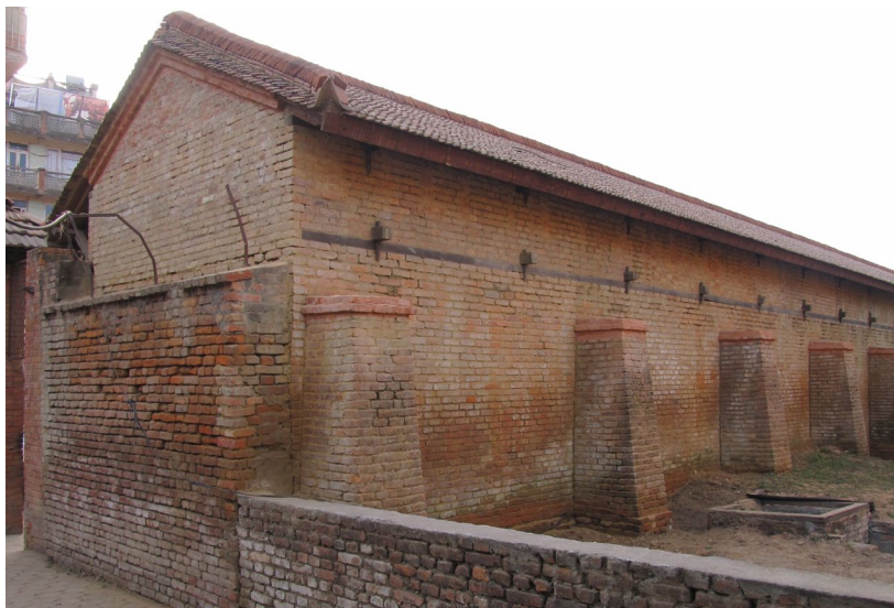
January 2013: Back façade and buttress walls after restoration.
