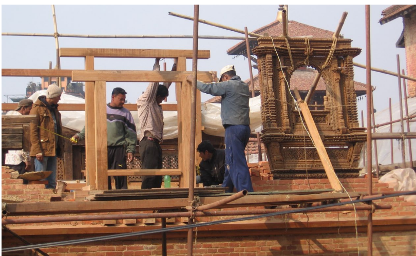
January 2011: Placing new inner window frames for the salvaged window brought from a house in Sundhara, Patan.
