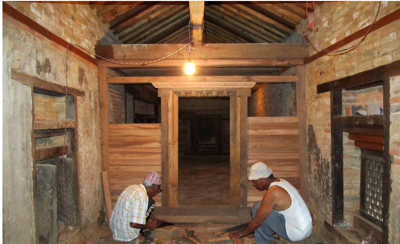
September 2012: Building a timber partition on the first floor of the west wing.
