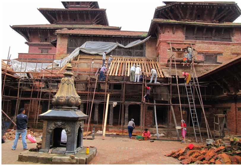
September 2011: Installing new timber joists on the north wing roof.
