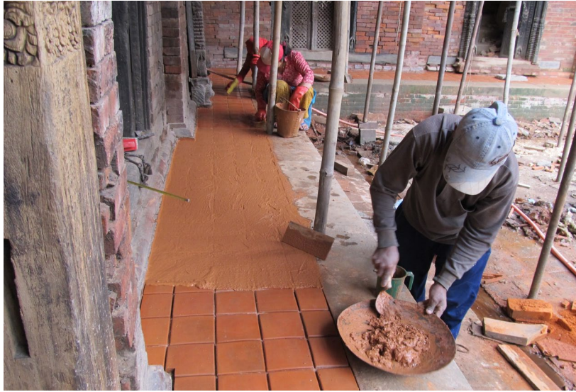
September 2011: Applying lime and brickdust ( surkhi ) grout after installing traditional chikah-apa floor tiles on the plinth.
