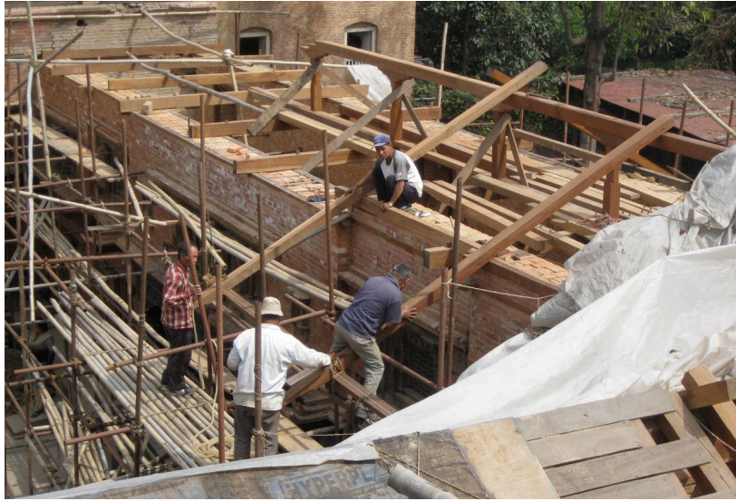
March 2011: Installation of roof timber structure on the east wing.
