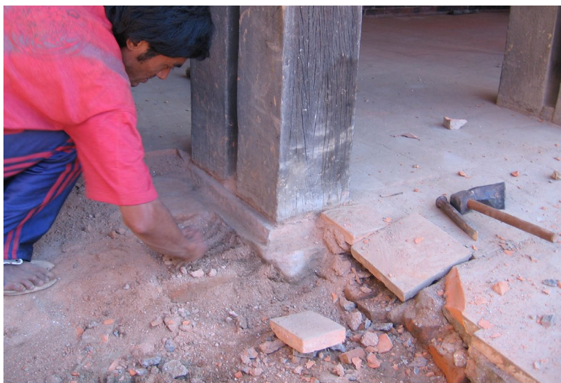
December 2012: Removing the old plinth pavement that covered the stone bases of the pillars.
