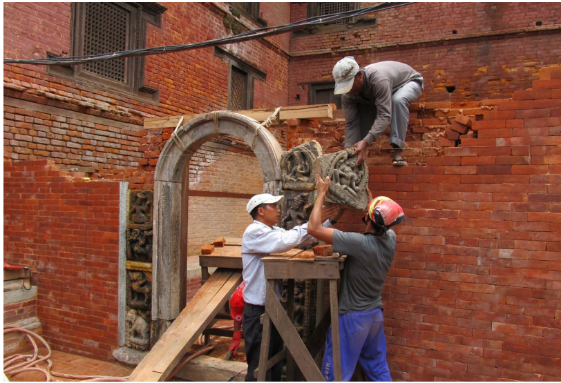
June 2012: The gate was rebuilt using the repaired stone statues and traditional bricks in lime and brickdust ( surkhi ) mortar.
