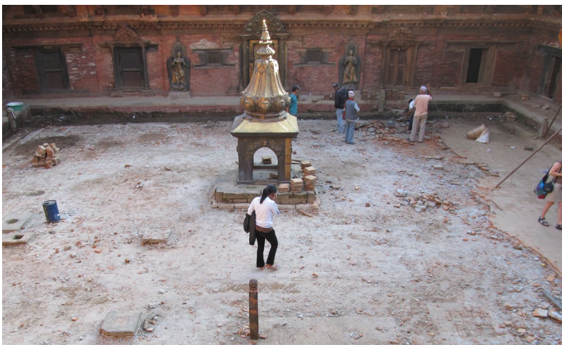
January 2012: Courtyard during excavation.
