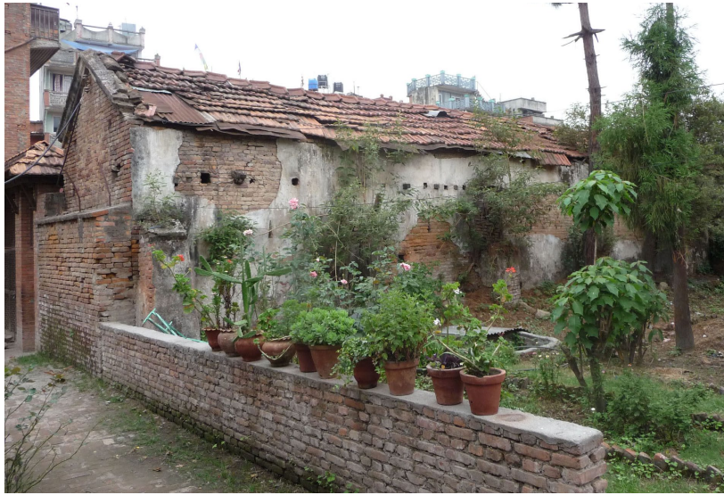
June 2009: Back façade of Kot Pati before restoration.
