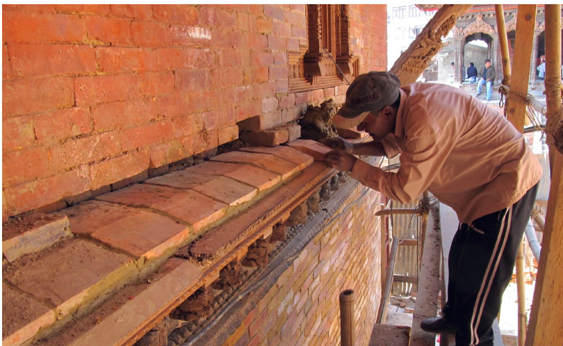
March 2012: Mason building brick cornice over timber cornice.
