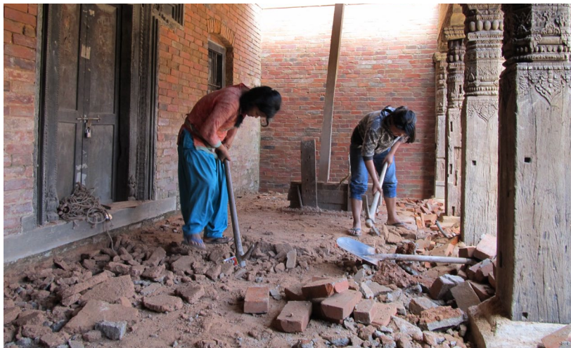
July 2011: Floor levels of the rooms north of the arcade on the north wing were lowered to match the historical level.
