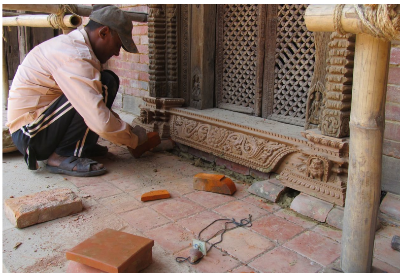
May 2012: New door jamb bases were installed where old ones were missing.
