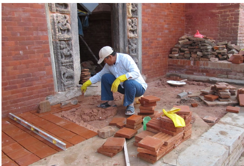
November 2012: Installing floor tiles ( chikah-apa ) in lime surkhi mortar in front of the gate.
