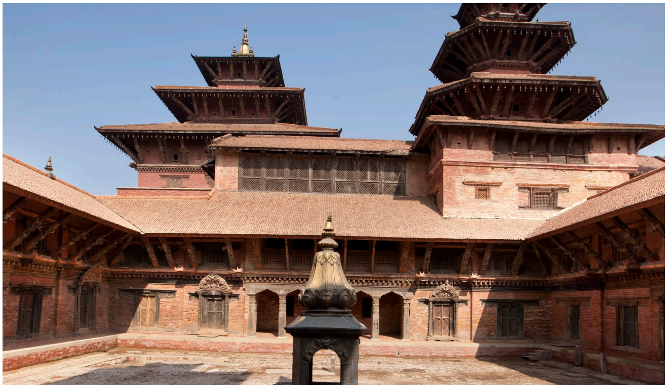
October 2006, December 2012: The courtyard façade of the east wing of Mul Chowk before and after restoration. Taleju Temple, at right, was structurally reinforced.
