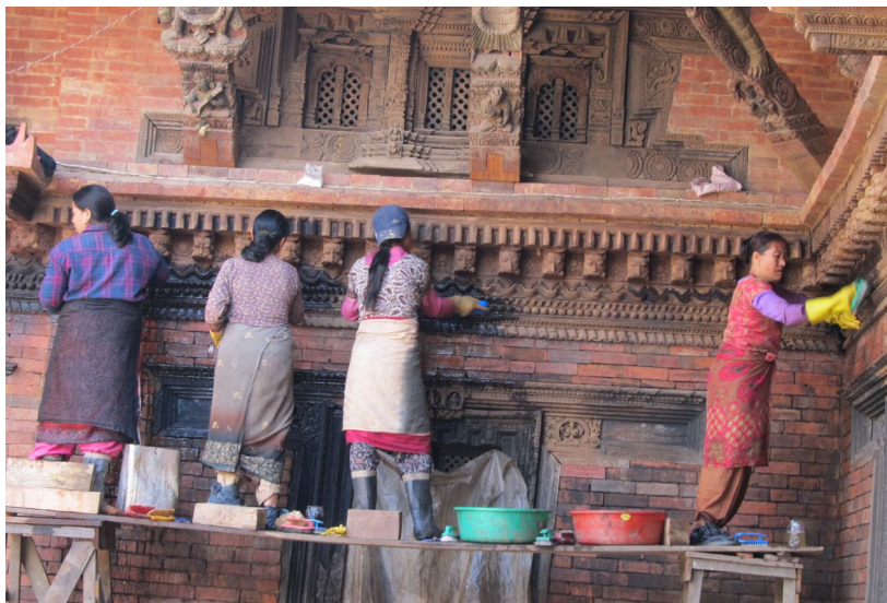
December 2010, September and October 2011: Removing black paint from pillars and cornices using water and caustic soda.
