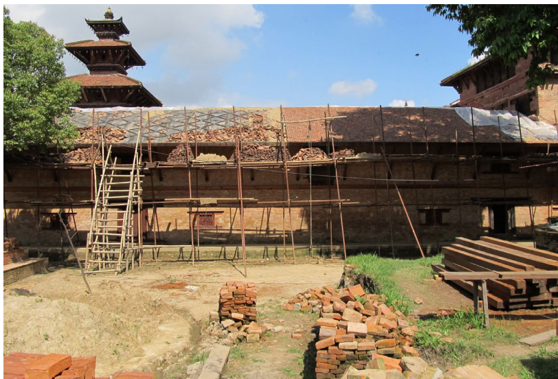
July 2011: East façade of the east wing during installation of roof cover.
