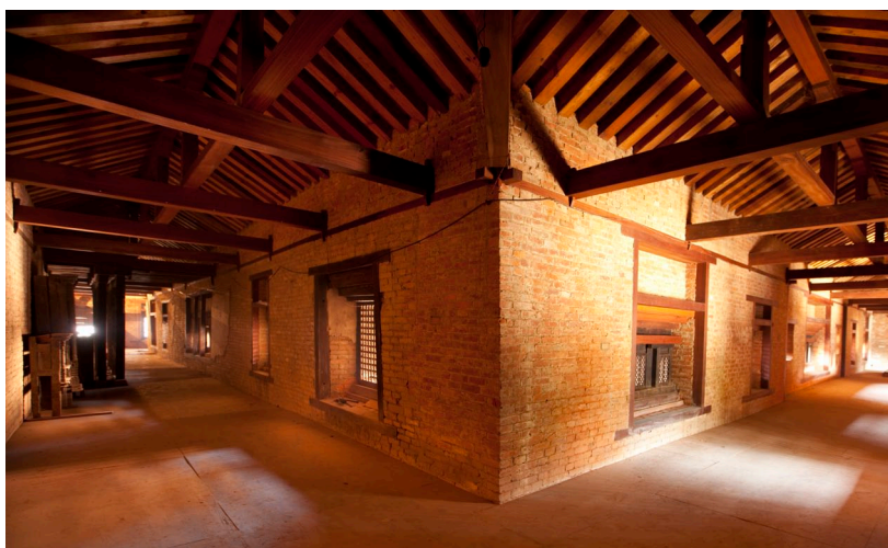
December 2012: First floor halls shortly after restoration.
