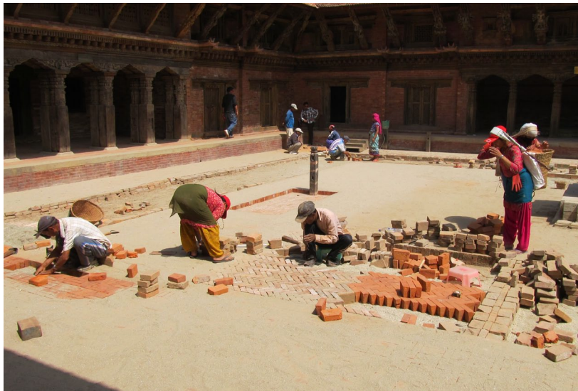
March 2012: Installing brick on-edge pavement in the original pattern using reusable historic bricks and matching new bricks.
