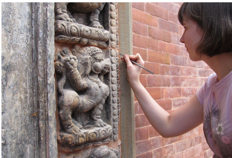
August 2012: Stone conservators from the University of Applied Arts Vienna applied the finishing touches to the restored sculptural elements.
