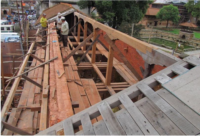
August 2012: Reconstruction of the Pati's roof structure after dismantling the existing, damaged timber elements.
