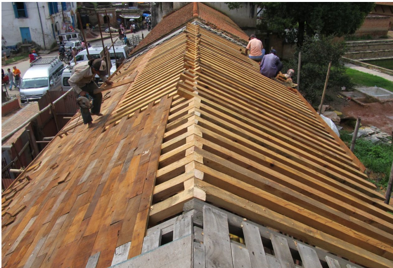
August 2012: Installing hardwood and plywood planking over the rafters.
