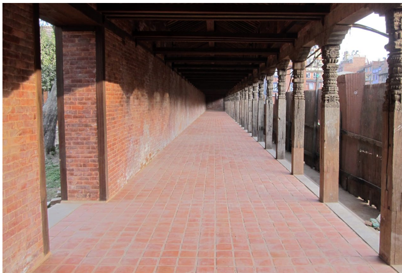
November 2012: View of the newly restored arcade and ceiling rafters.
