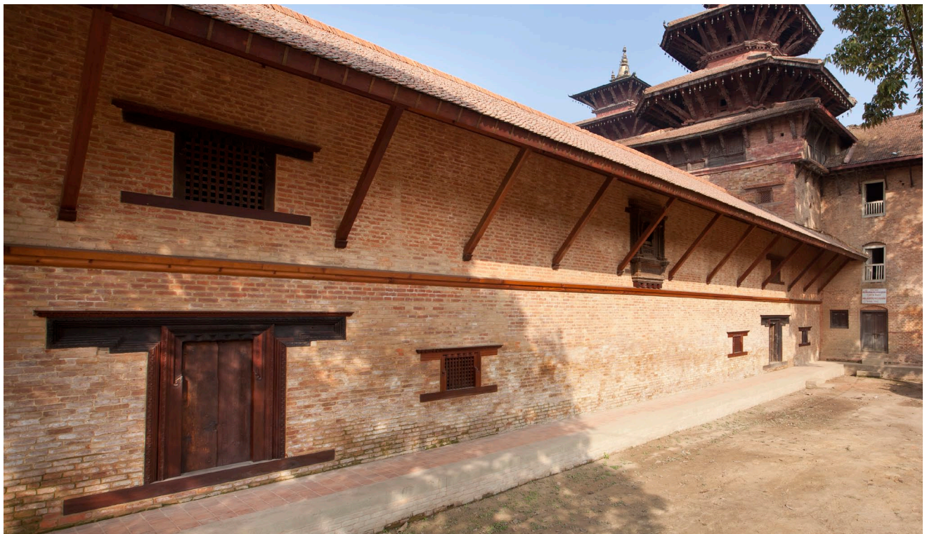
May 2006, December 2011: The east façade of the east wing of Mul Chowk before and after restoration.
