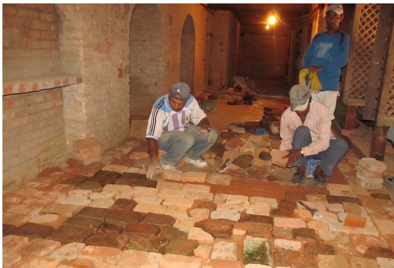
July 2012: Brick soling in lime surkhi mortar being applied over the timber floor structure.
