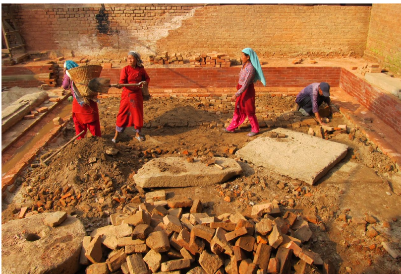
March 2012: Debris was removed from site, and flat brick soling was done on the courtyard.
