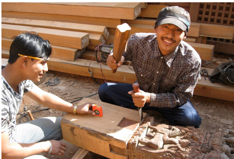
October 2011: Grafting on an extension to a damaged roof strut, employing a cross-joint.
