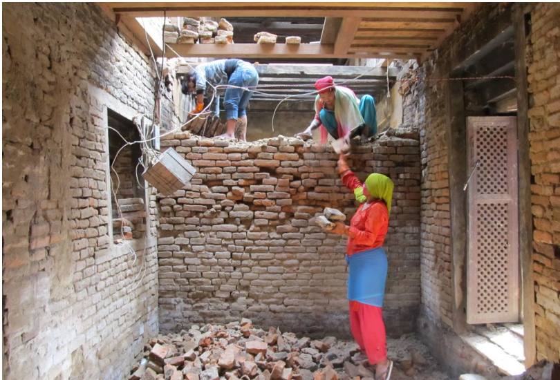
August 2011: Dismantling the dilapidated partition wall on the west wing.
