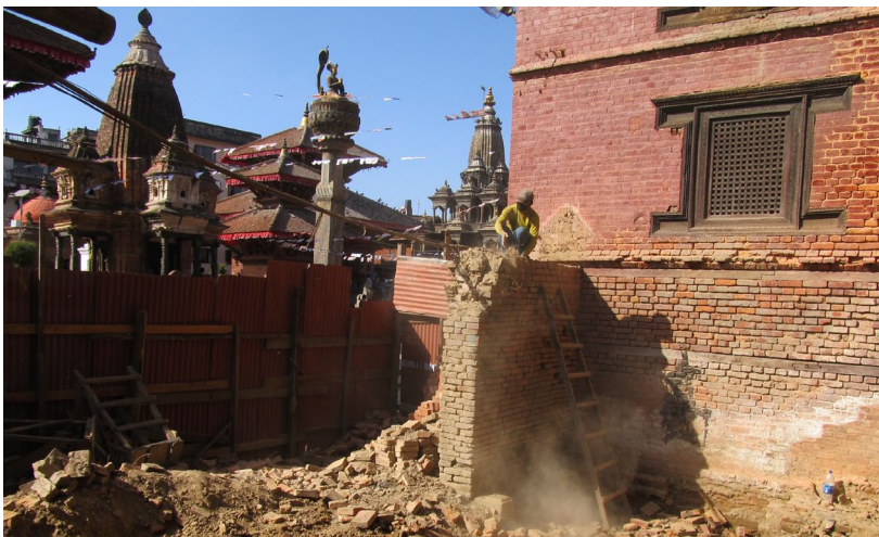
February 2012: The badly damaged courtyard wall surrounding the south Stone Gate was demolished
