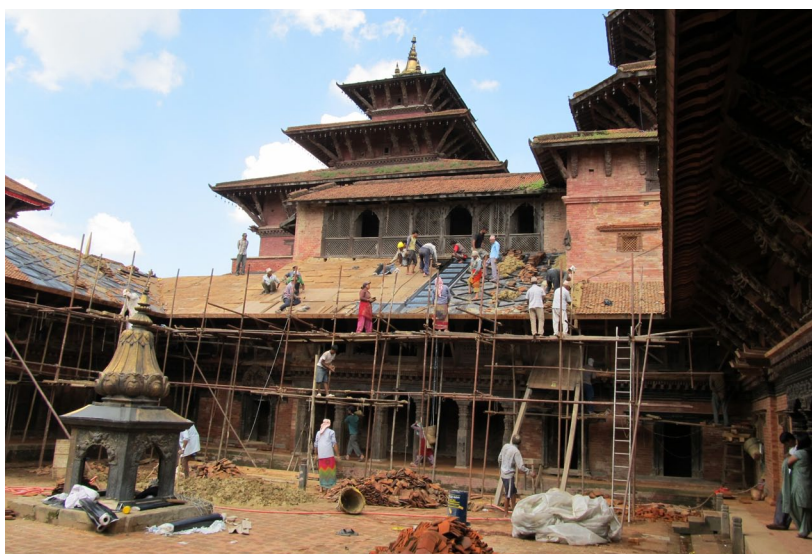
September 2011: Placing a waterproof membrane over the hardwood planking.
