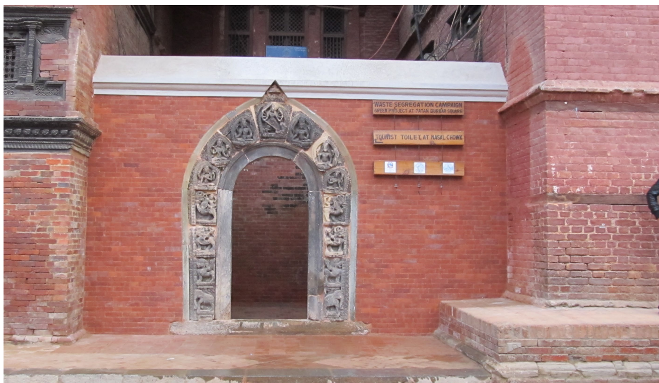
July 2012, November 2012: North stone gate before and after restoration.
