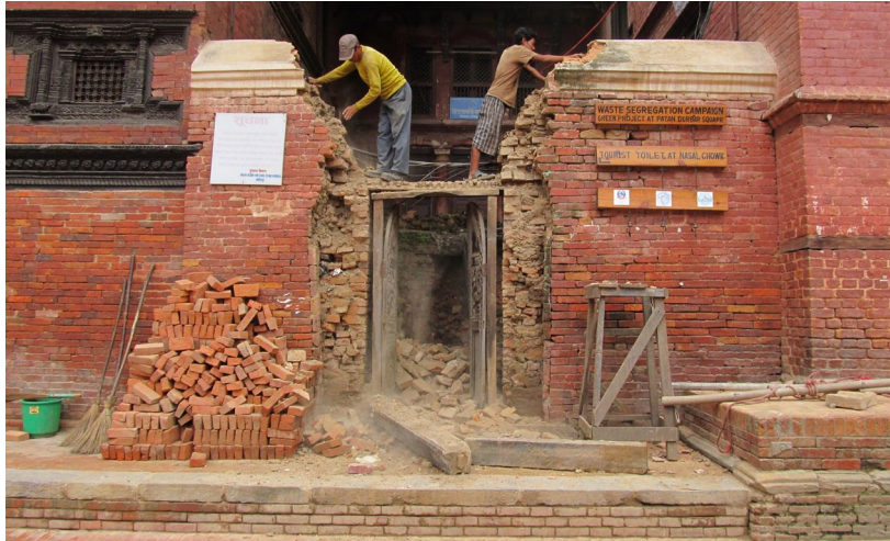
July 2012: Dismantling the dilapidated brick wall surrounding the stone gate.
