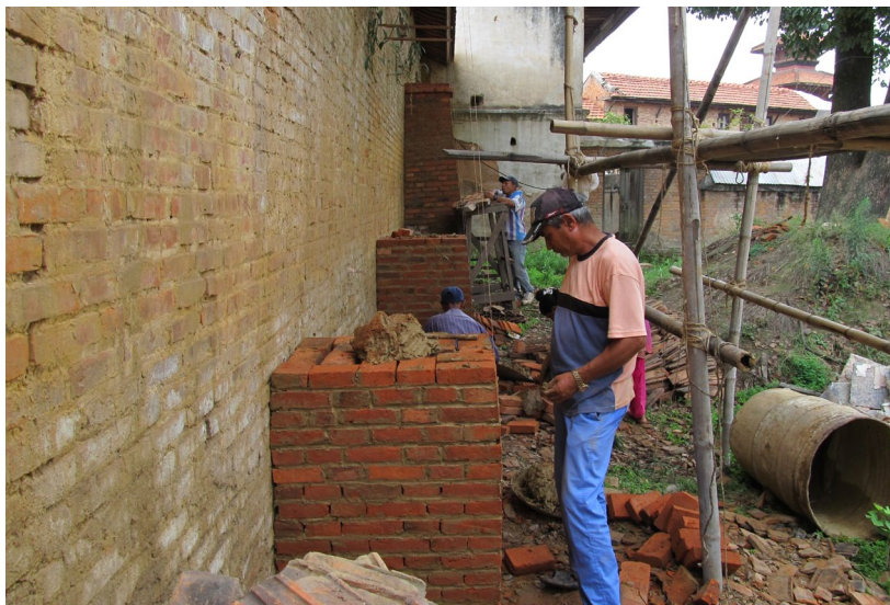
June 2012: Rebuilding the buttress walls using traditional ma-apa bricks.
