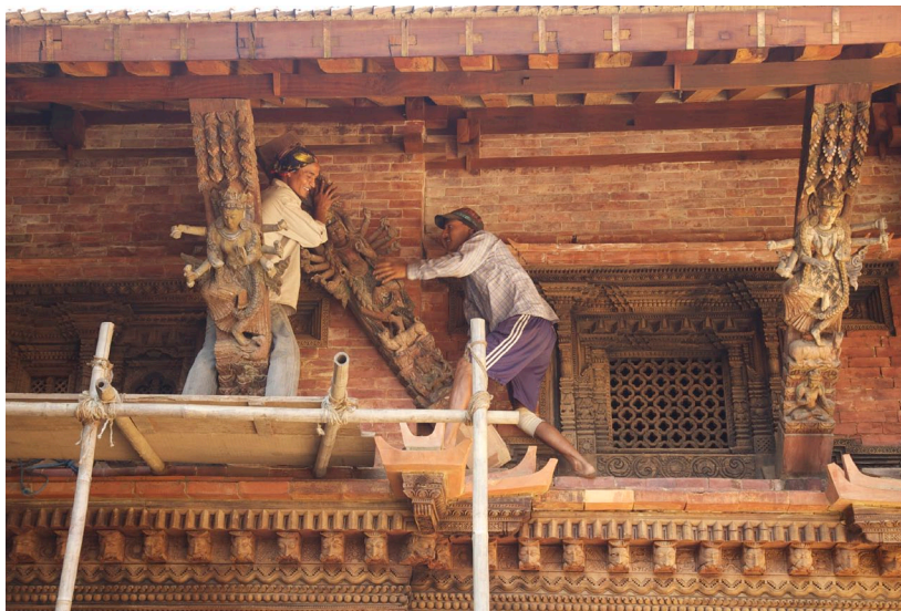
October 2011: Removing roof struts for cleaning and repair.
