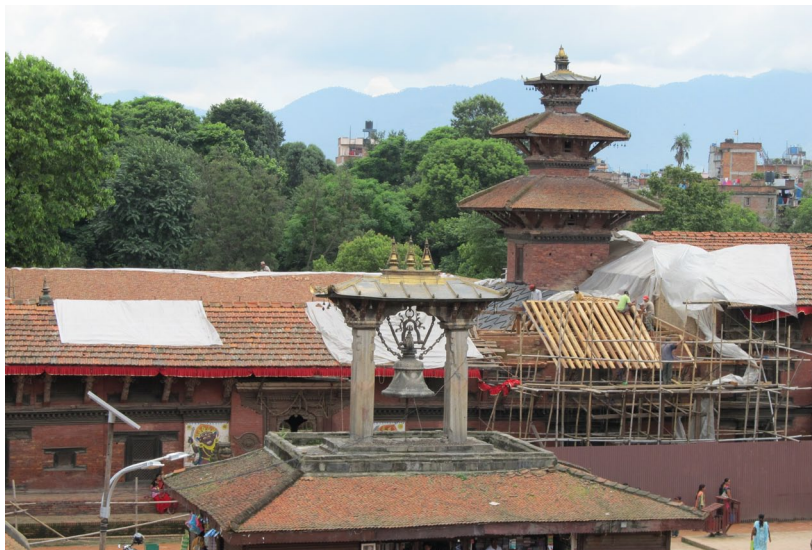
July 2011: Installing new timber joists on the west wing roof.
