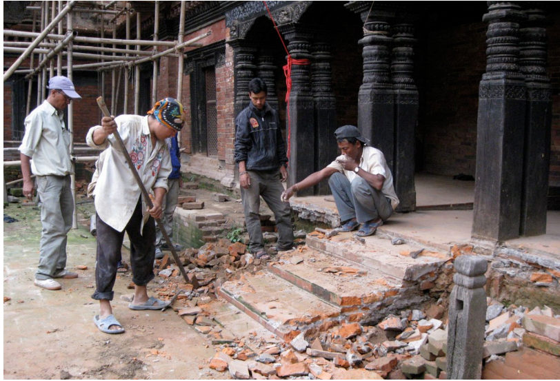
July 2011: Dismantling unhistorical paving, steps, and plinth.
