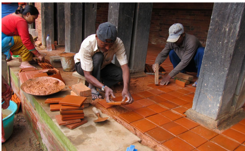
August 2011: Traditional floor tile chikah-apa were laid in lime and brickdust ( surkhi ).
