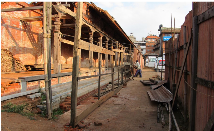
February 2012: The building was fenced when construction began.
