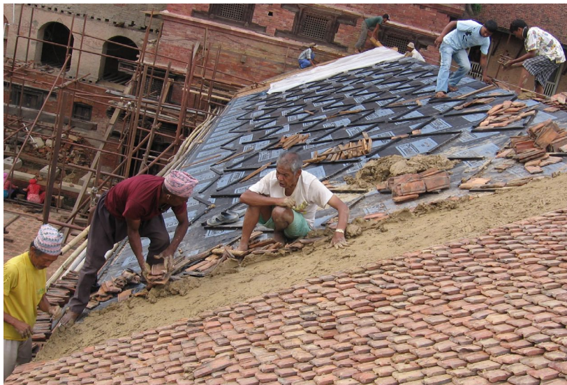
June 2011: Laying traditional roof tiles ( jhingati ) on a mudbed over the waterproof membrane on the east wing roof.
