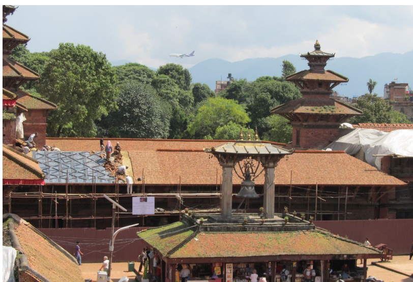
September 2011: Installation of traditional jhingati roof tiles on the west wing roof.
