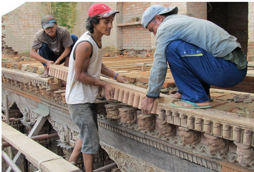
July 2011: Lost timber dental cornices were refabricated and installed above the lion heads using traditional timber joints.
