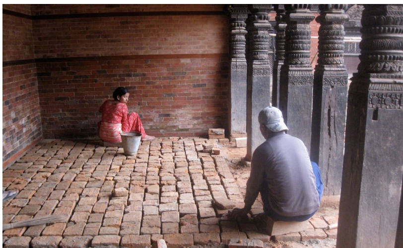
August 2011: Flat brick soling was installed on a sand bed.
