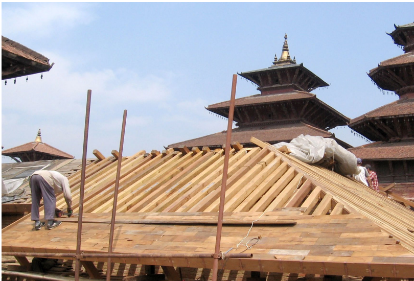
March 2011: Detail of sal hardwood planking on the south-east corner.
