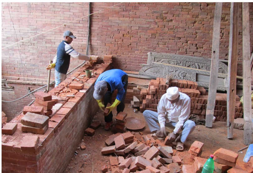
November 2012: Building the parapet wall.
