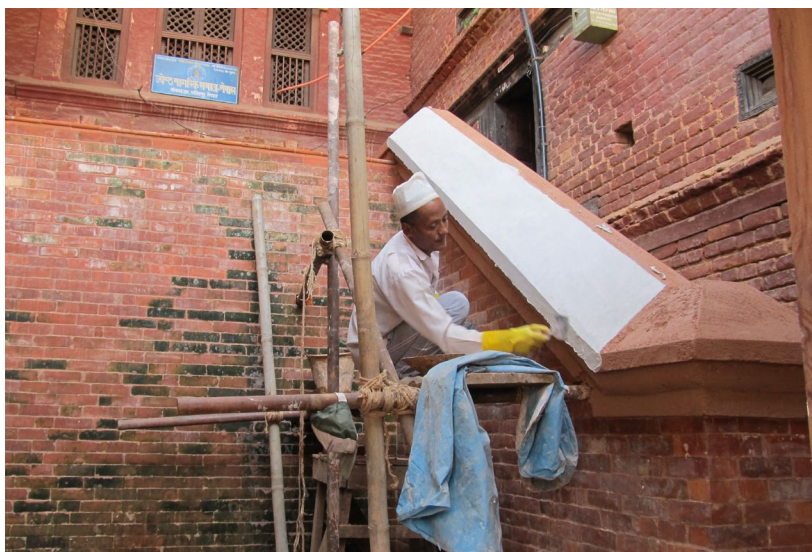
November 2012: Applying lime plaster to the parapet wall on the stone staircase.
