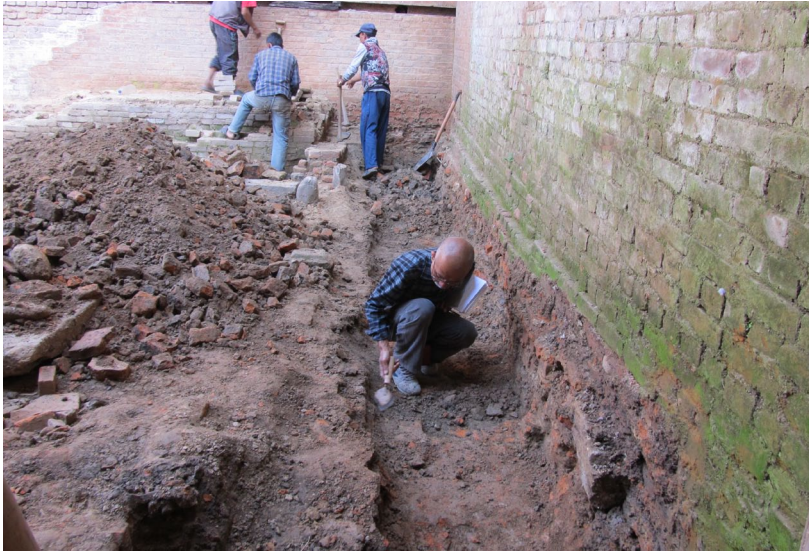
February 2012: Excavating the courtyard to remove the foundation of the existing dilapidated plinth.
