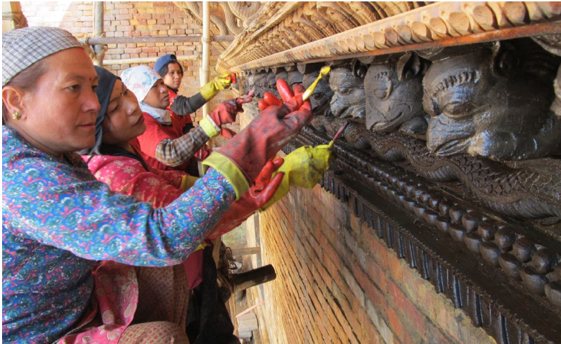
March 2012: Women cleaning existing timber cornice in-situ using plain water and caustic soda.
