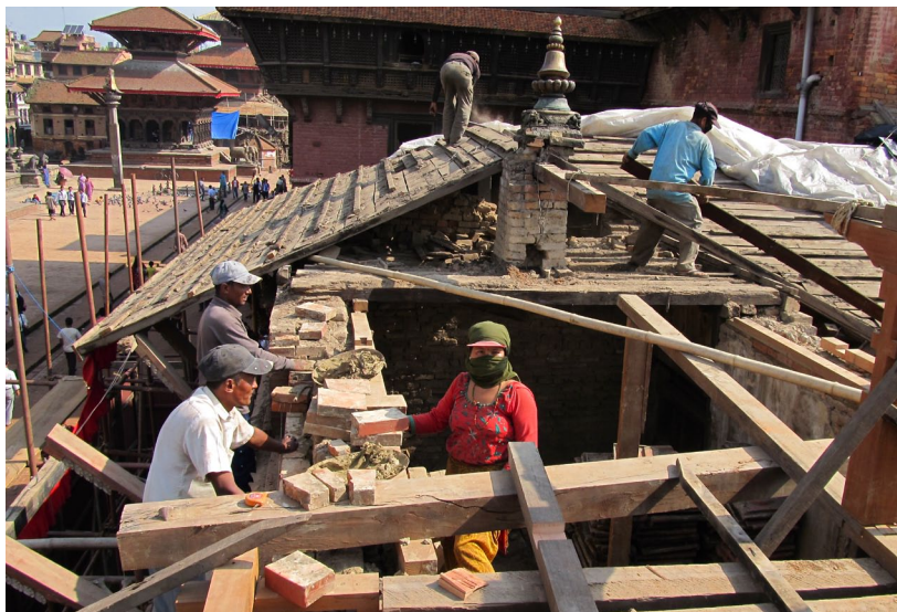
June 2011, August 2011: Removal of roof structure from the west wing.
