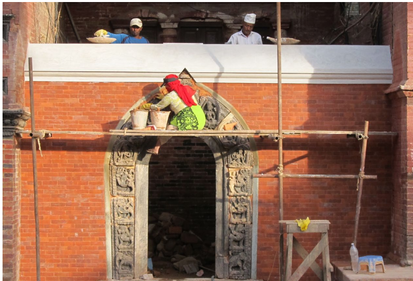
November 2012: Finishing the stone gate brick wall.
