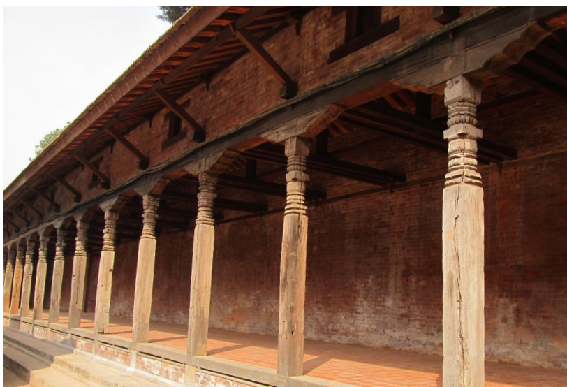
August 2012: Exterior frontal view of Kot Pati after restoration.
