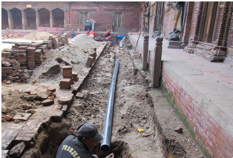
February 2012: Laying PVC pipes underground for installation of rain water drain.
