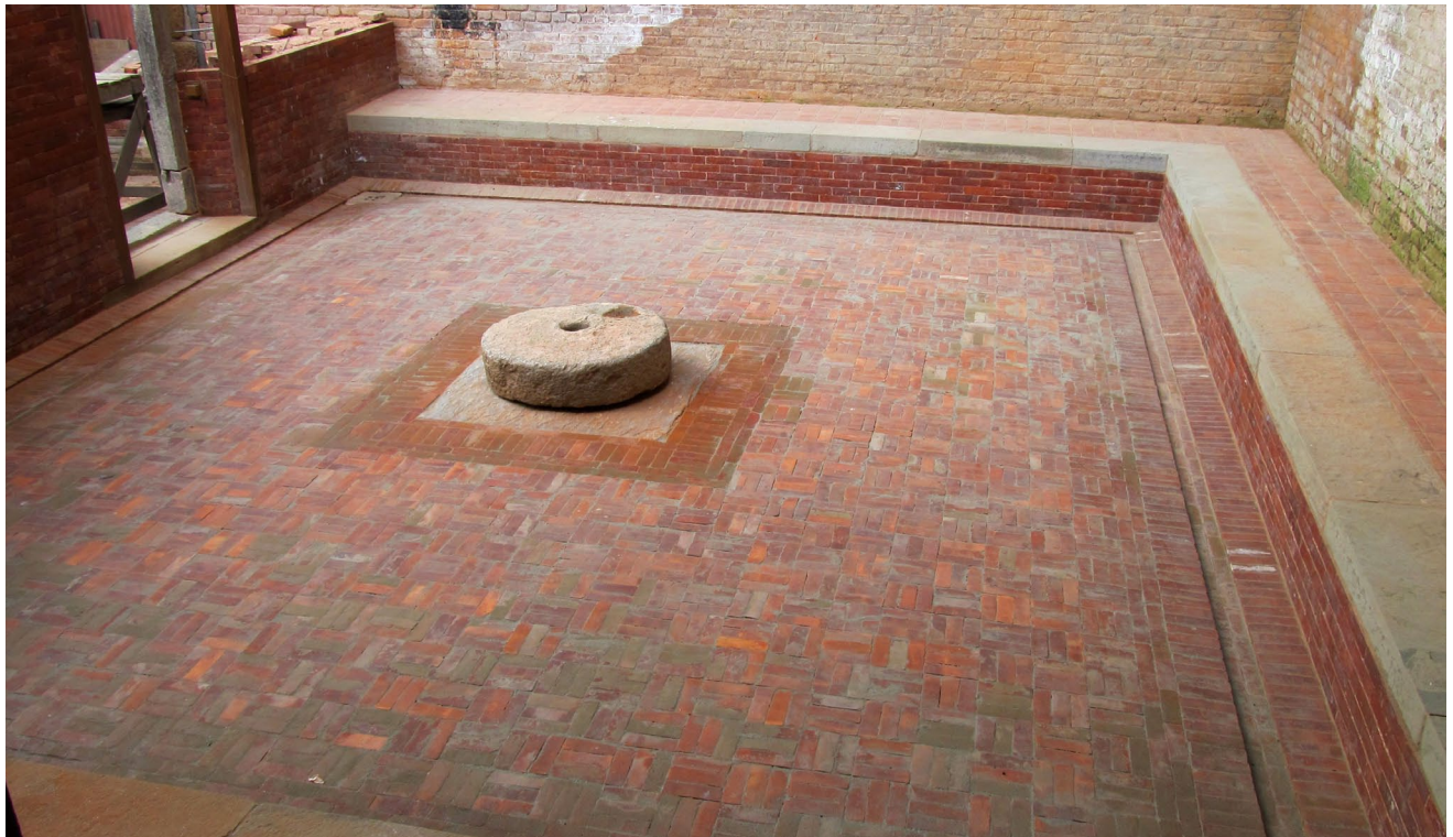
May 2012: Courtyard during installation of the brick on-edge pavement over a sand bed. A surface rain-water drain was installed along all walls.
