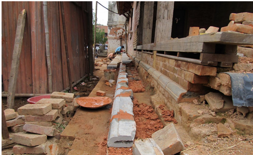
June 2012: The plinth was rebuilt with traditional edge stone and stone nagol (bead) in lime and brickdust ( surkhi ) mortar.
