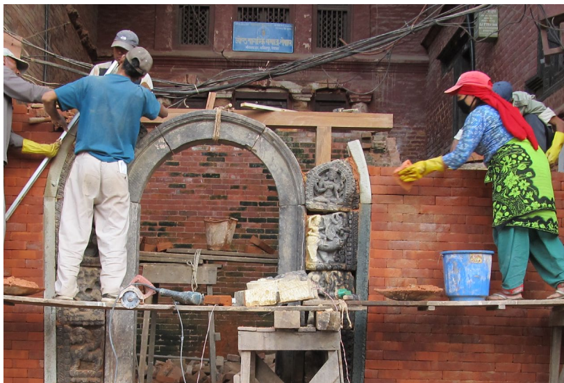
October 2012: The gate was rebuilt using existing stone statues and traditional bricks in lime and brickdust ( surkhi ) mortar.
