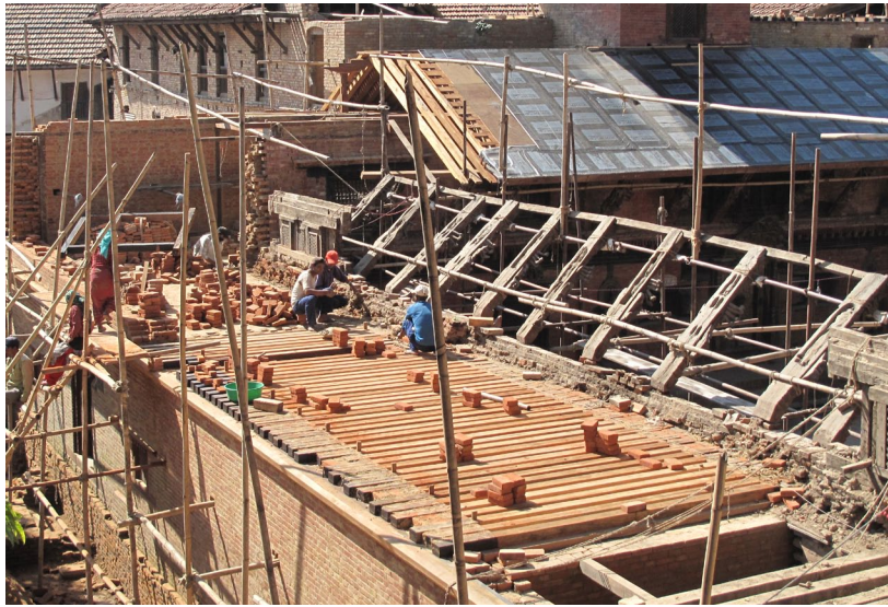
November 2010: Installing new timber floor structure on the east wing first floor.
