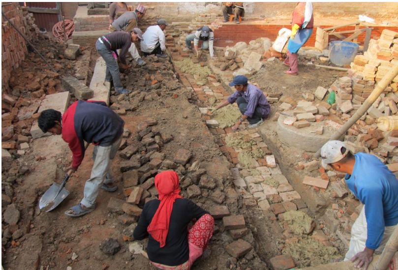
March 2012: The foundation of the principal wall running along the Darbar Square was excavated and built up again to ground level using yellow mud mortar.
