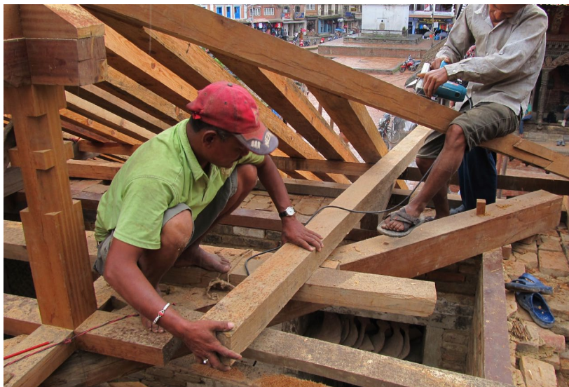
September 2011: Detail of traditional timber joinery for the roof structure on the northwest corner.
