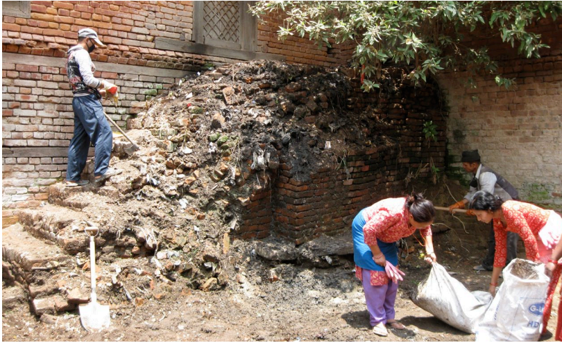
May 2011: The courtyard filled with junk was cleaned before restoration began.
