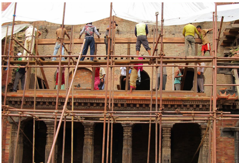
July, August, September 2011: Rebuilding the north wing façade.
