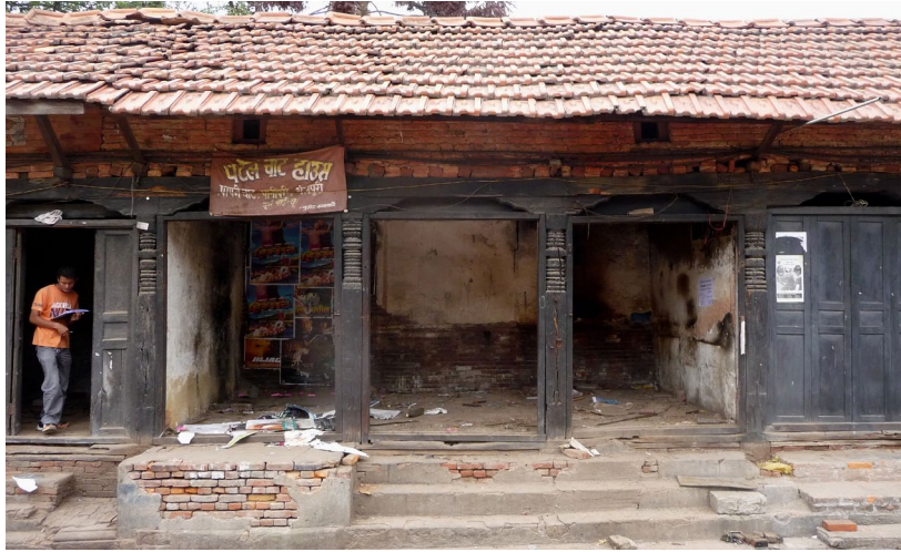
June 2009: Existing front and back elevations of Kot Pati before restoration.
