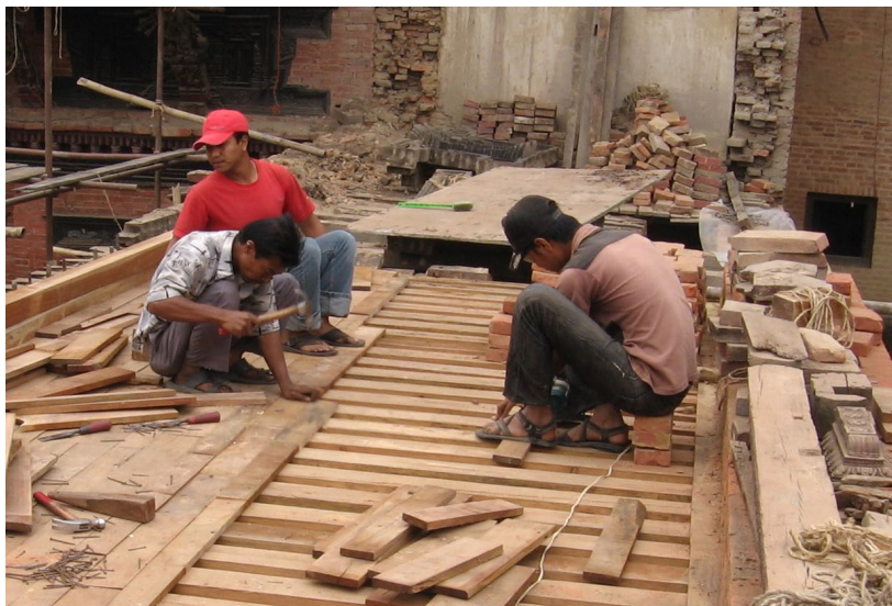
January 2011: Sal /hardwood planking being placed over the floor joists.
